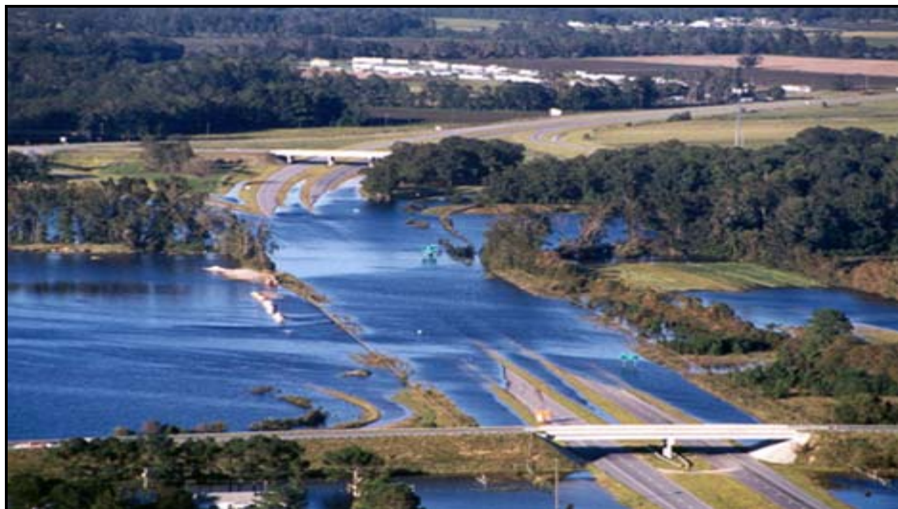
Image 4: Flooded View of Highway 264 Bypass
