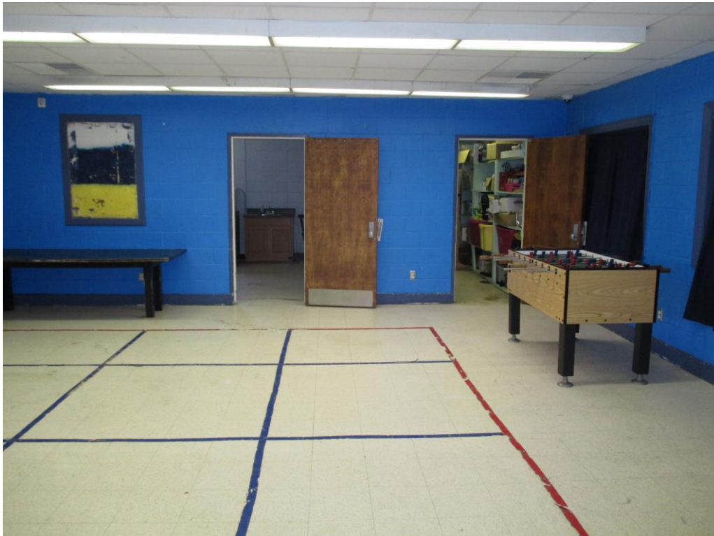
Photo 4 View across the kid's area. Showing floor tile observed in this area. The mastic under the floor tile in this area is positive for asbestos.
