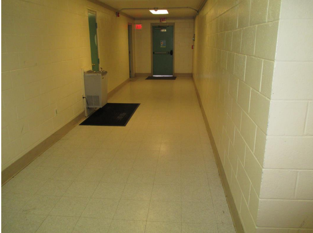
Photo 8 Typical view of the floor tile and cove board in the hallway area. There were two layers of floor tile (the visible top layer and a second layer underneath the visible layer) in the hallway areas. Both layers of tile and mastic associated with both tile layers are negative for asbestos.
