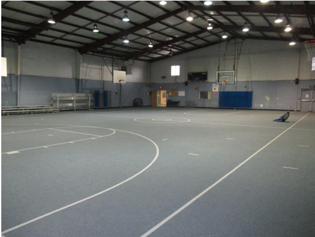
Photo 1 Typical view across the gym. Showing the blue carpet covering the gym floor. Floor tiles under this carpet were positive for asbestos.
