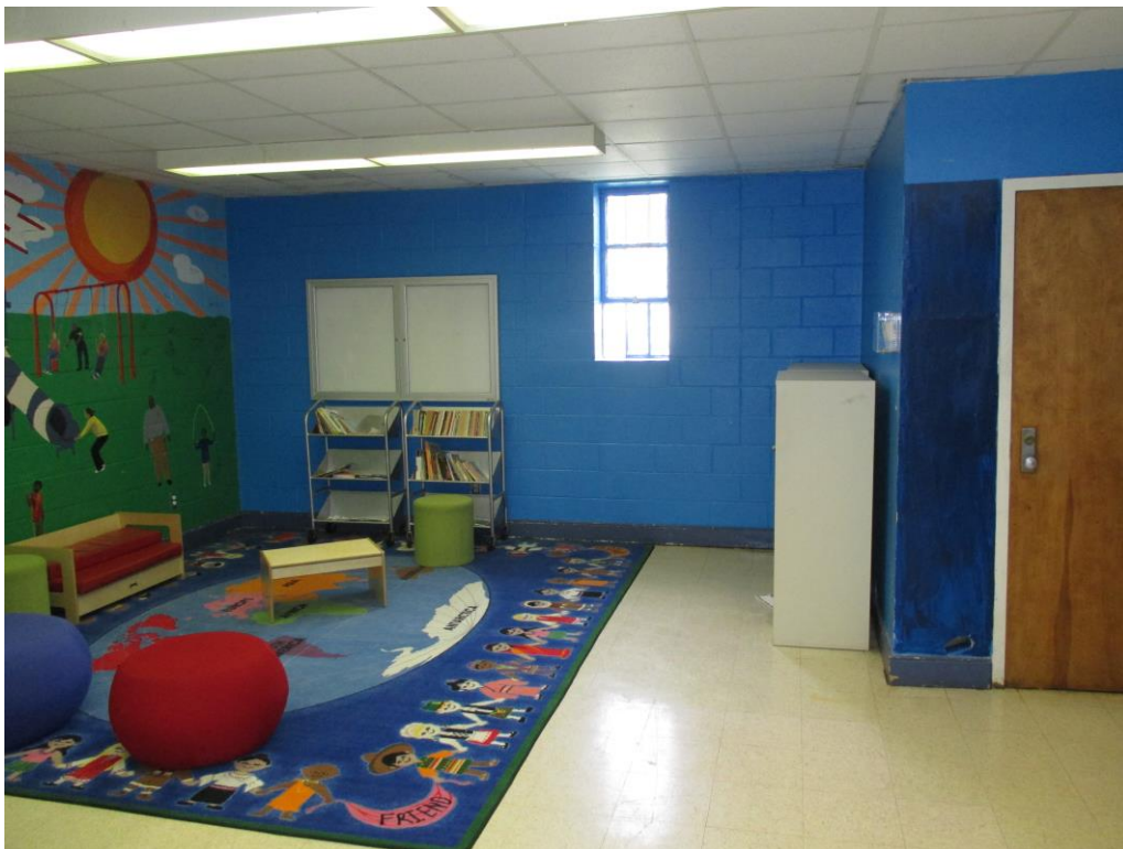
Photo 6 An additional view across the kid's area. Showing a window commonly observed in the building.
