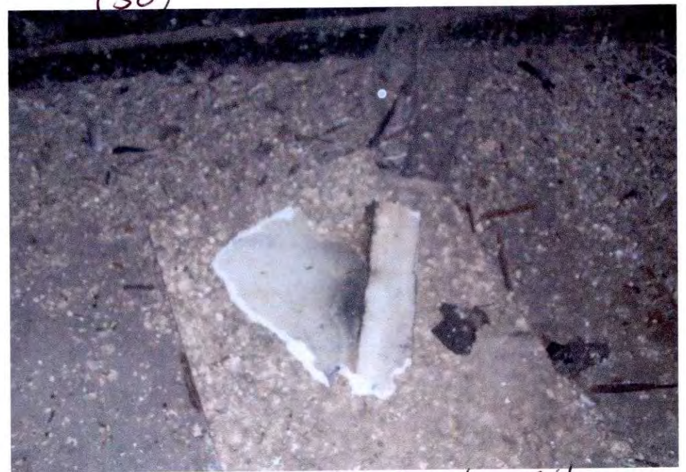
Asbestos panel in side Bldg.
