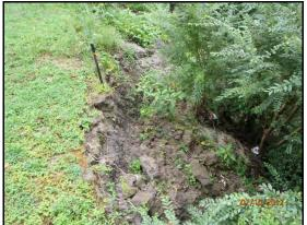
Picture 5-5. Left bank erosion adjacent to residential lawns without stream buffer
