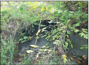
Picture 4-4. Obstruction at Tucker Drive Culvert Crossing (Meetinghouse Branch)
