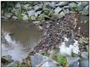
Picture 5-3. Existing rock drop structure
