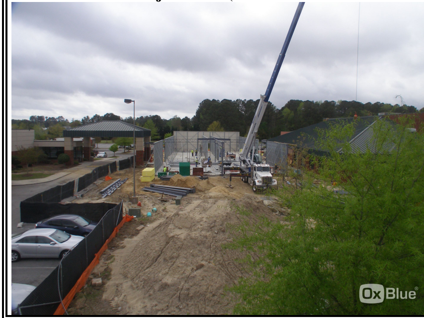
Current Photo of Project Area: (Greenville Convention Center Renovation and Expansion)
