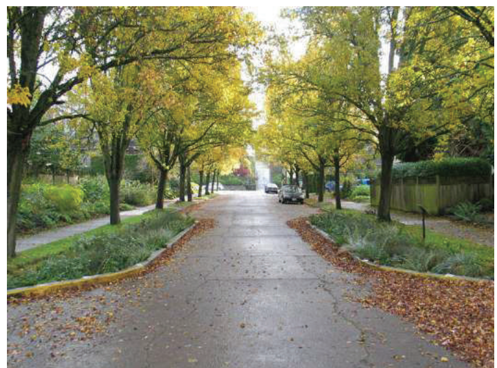
Bioretention Traffic Calming
