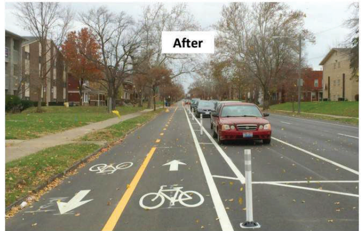
Street Resurfacing and Restriping
