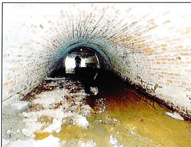
Culvert Section 2 looking downstream
