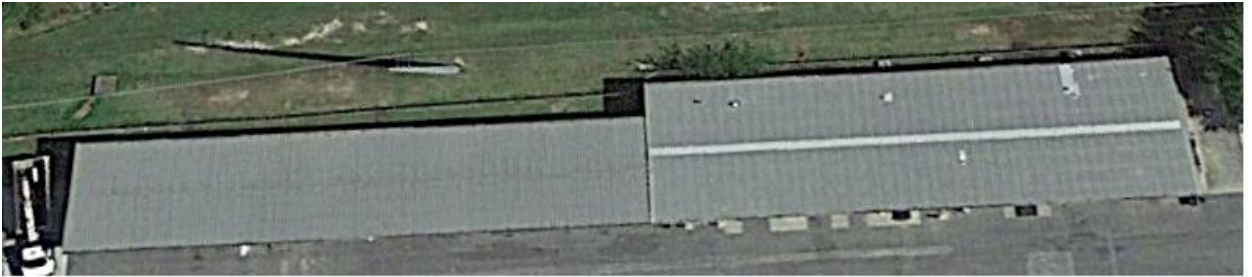
Building D – Streets Maintenance Division
