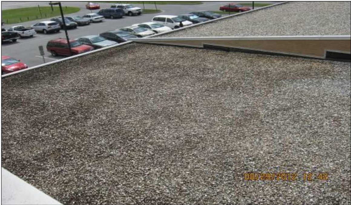
Overview of Roof Area D
