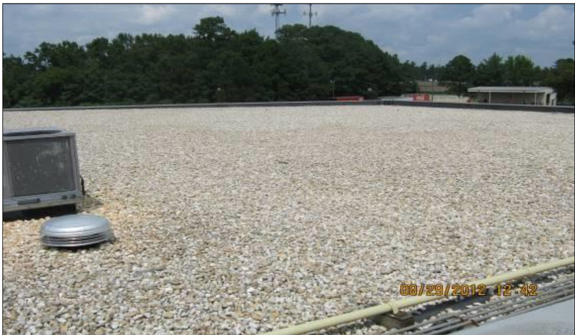
Overview of Roof Area C
