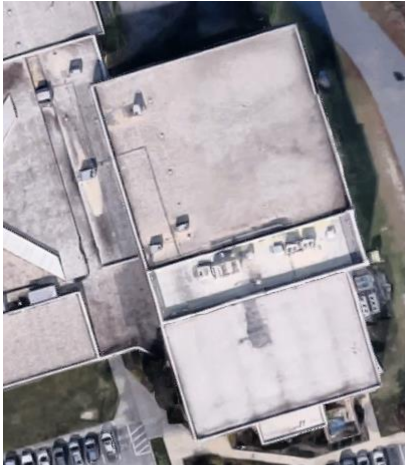
Overview of Roof
