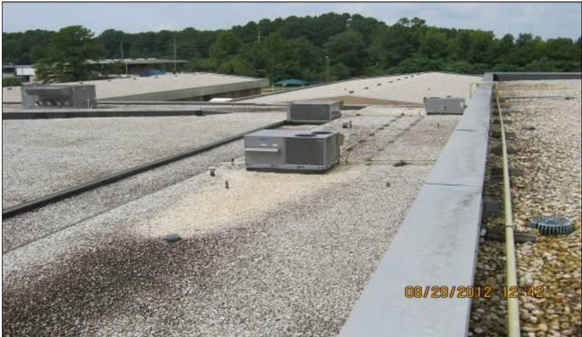
Overview of Roof Area E & F
