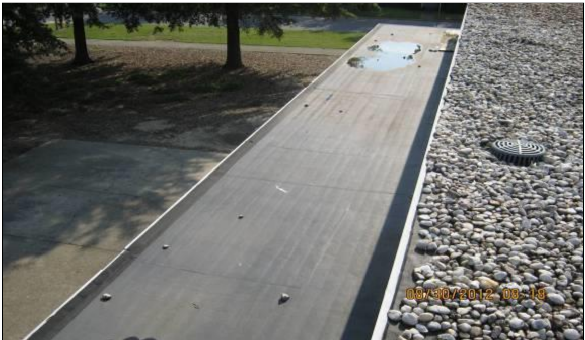
Overview of Roof Area E
