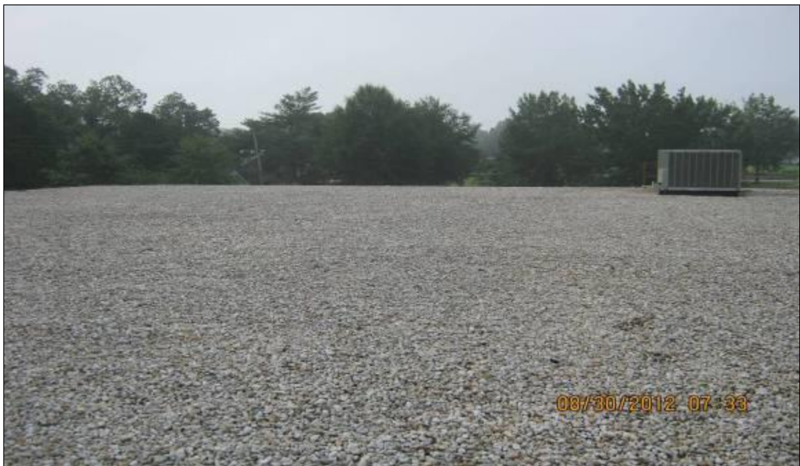
Overview of Roof Area A
