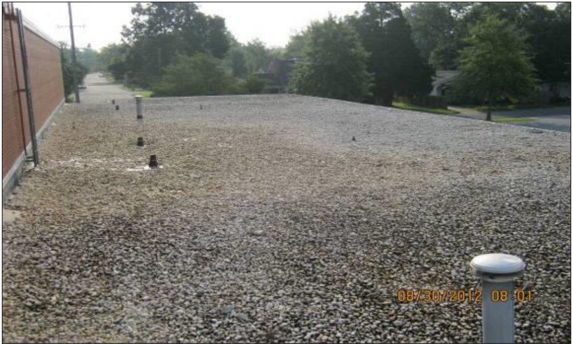
Overview of Roof Area D
