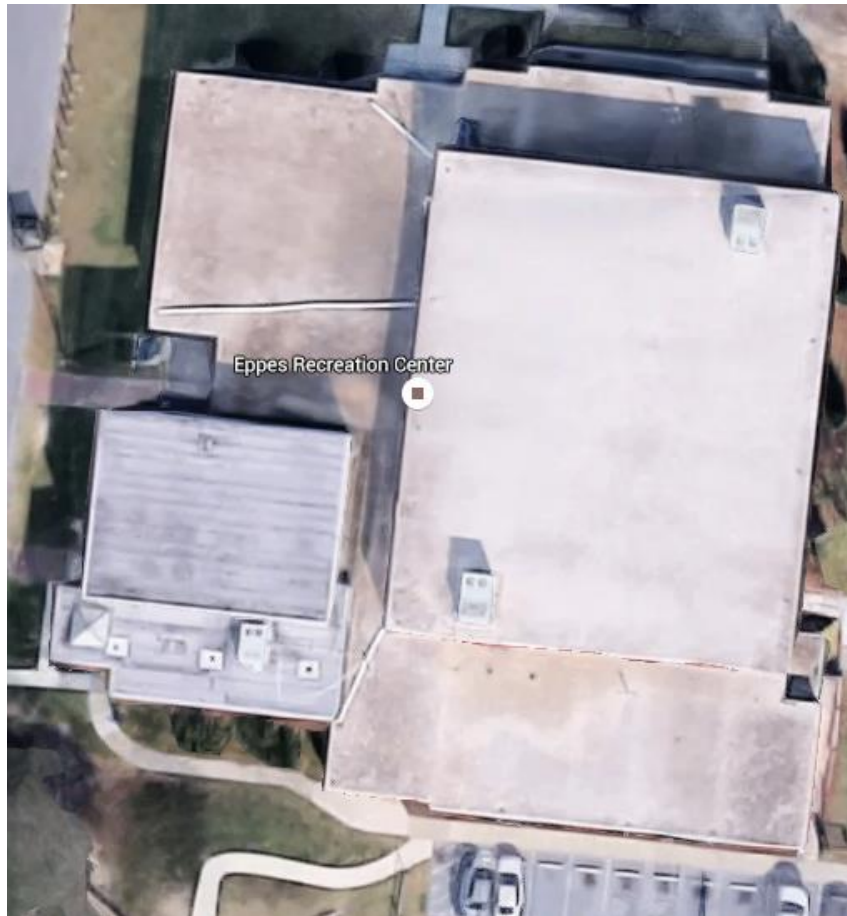
Overview of Roof
