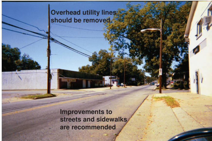
View west on Martin Luther King, Jr. Drive
