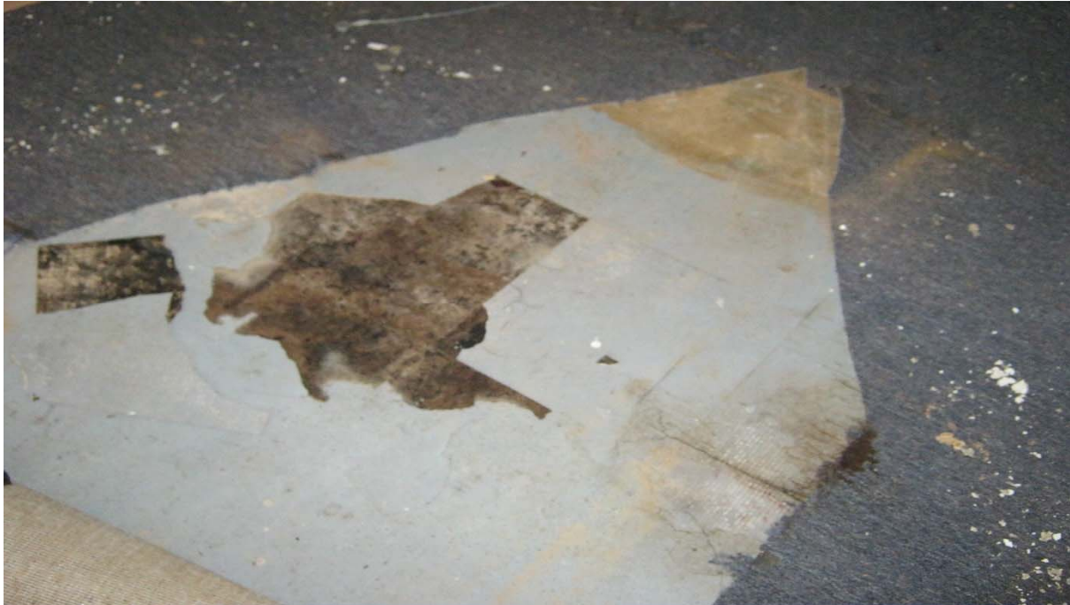
Floor Tile Mastic underneath 12" floor tile and carpet throughout the space.
