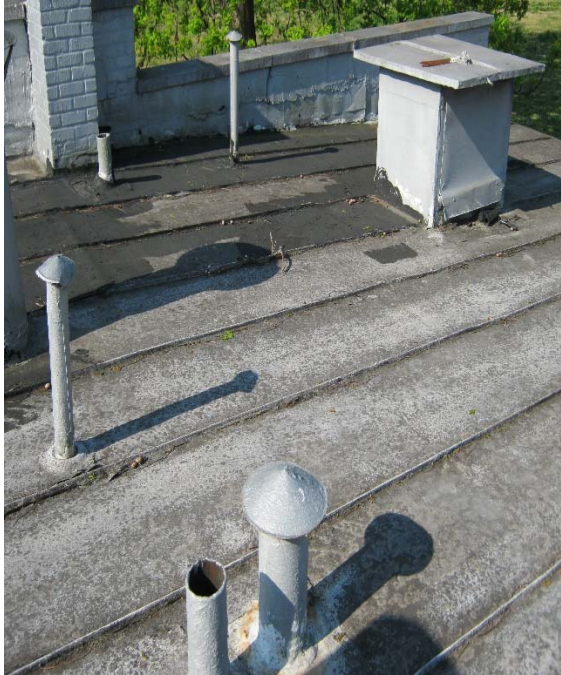
Cool Seal / Tar on Penetrations and Chimneys
