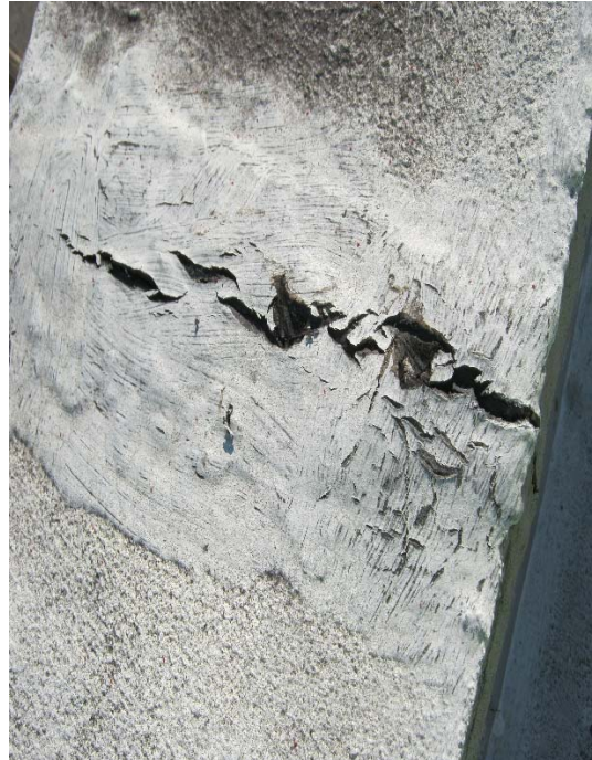
Sealant on Parapet Wall Seams and Cracks.
