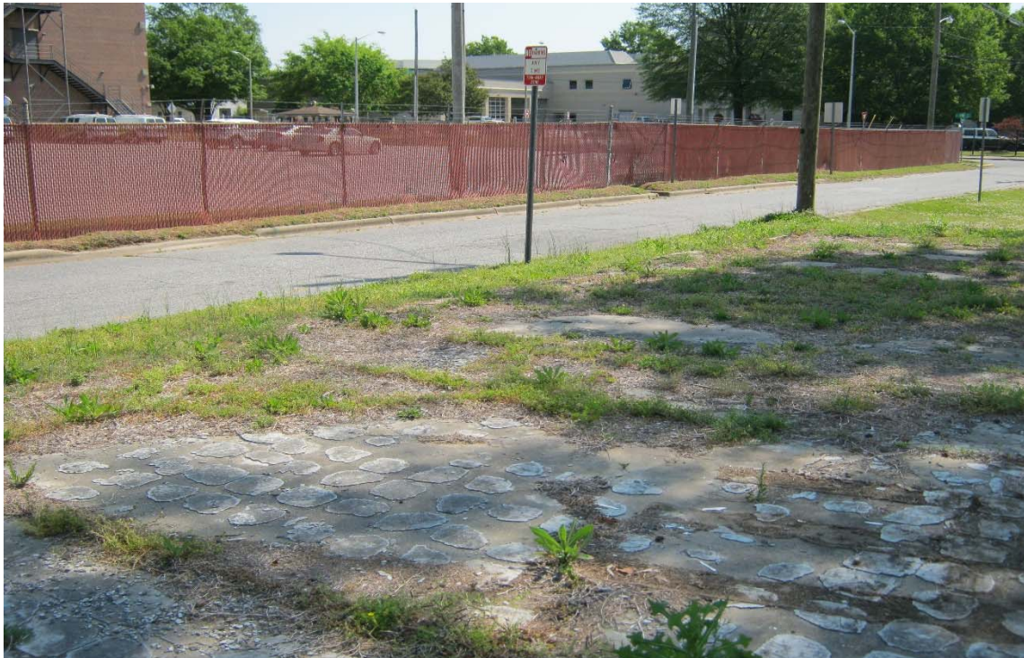
Remaining floor tile on the right side of the empty concrete pad.
