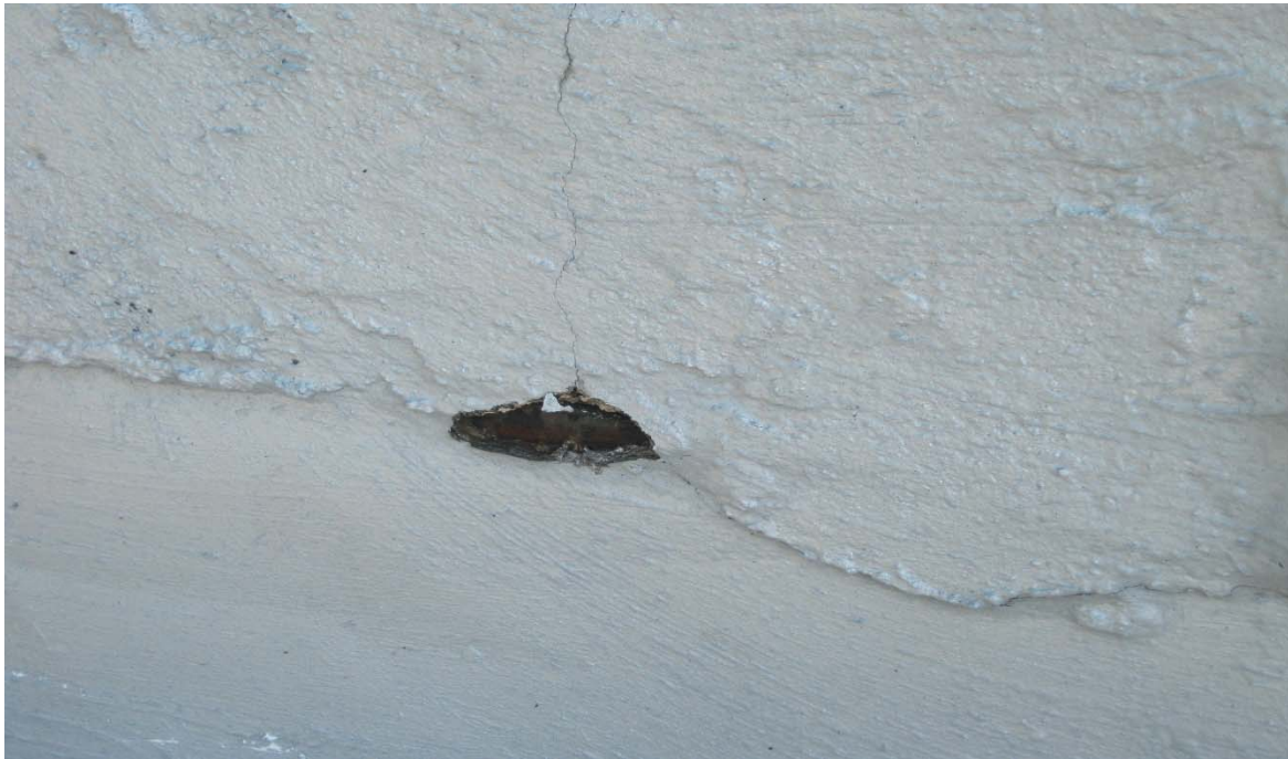
Skim / Cool Seal on Brick Parapet Walls.
