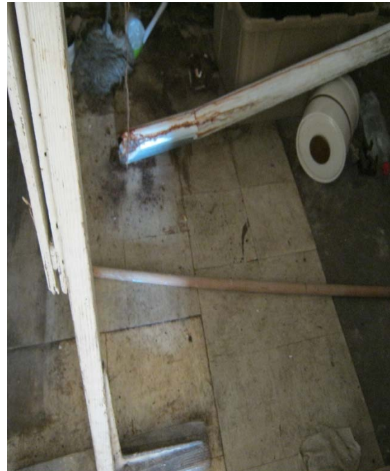
9" Floor tile and mastic in rear area.
