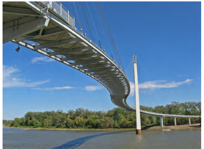
Bob Kerry Pedestrian Bridge between Omaha, NE and Council Bluffs, IA
