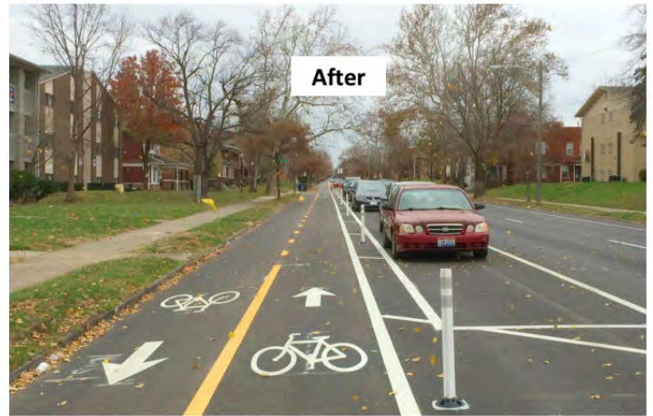
Street Resurfacing and Restriping
