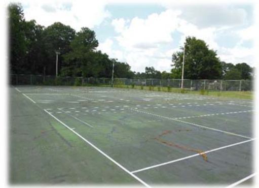
Tennis Courts at Jaycee Park.
