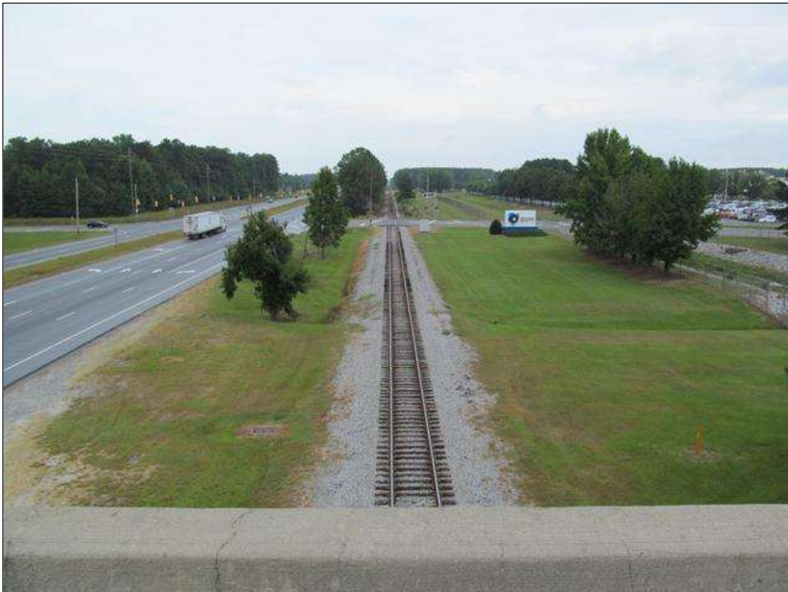
LOOKING NORTH, CSX RAILROAD.
