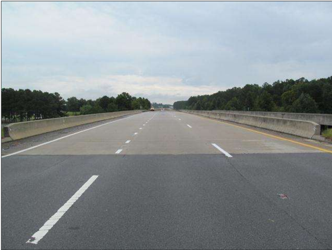
LOOKING EAST, US264 WEST BOUND LANES.
