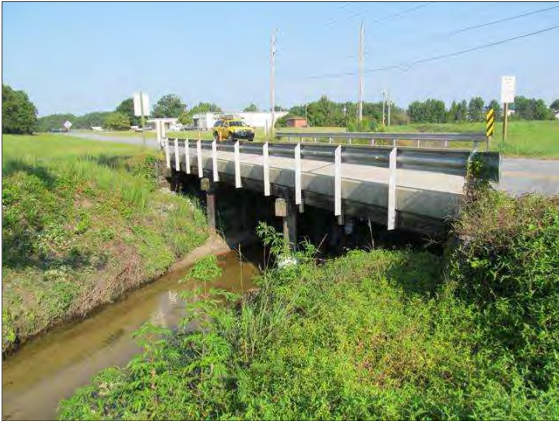
SOUTH SIDE, LOOKING WEST
