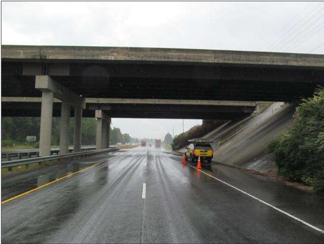
SPAN 1 CLEARANCES, LOOKING SOUTH US13/NC11/NC903.
