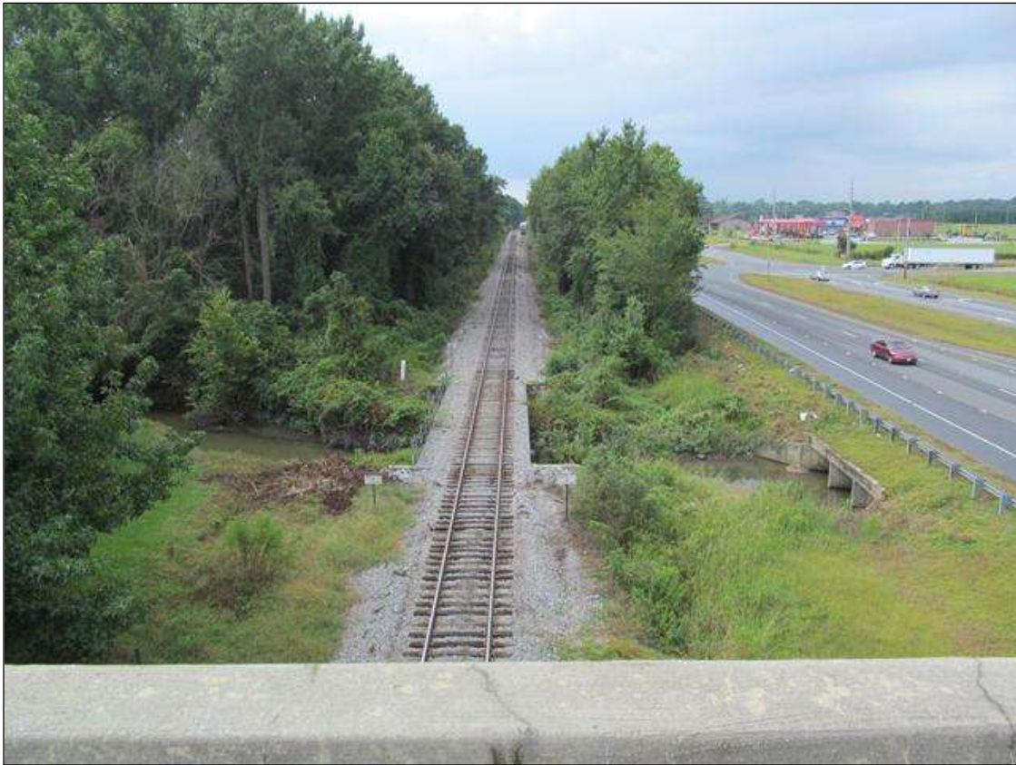
LOOKING SOUTH, CSX RR
