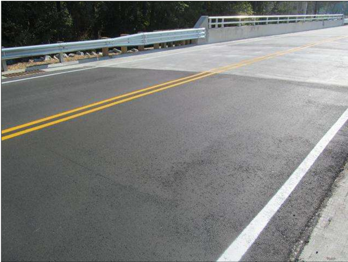
WEST APPROACH WEARING SURFACE WITH NO NOTEWORTHY PROBLEMS. EAST APPROACH SIMILAR.
