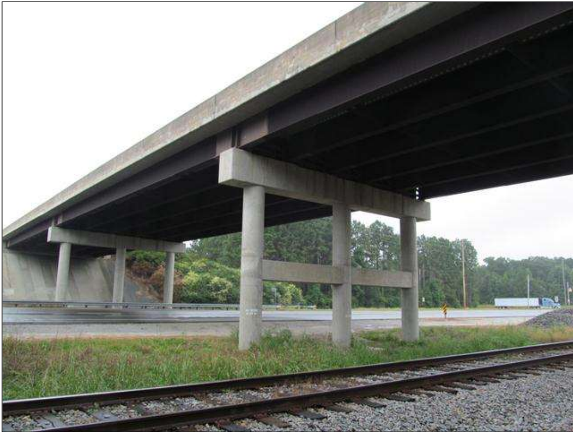
SOUTH SIDE, LOOKING WEST.
