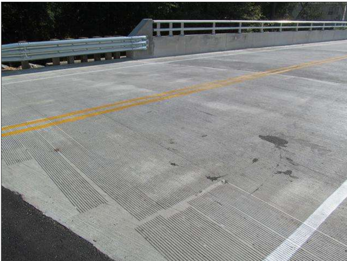
WEST APPROACH SLAB. EAST APPROACH SLAB SIMILAR.
