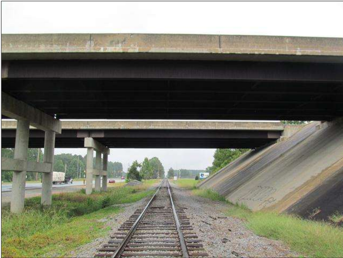
SPAN 3 UNDERCLEARANCE, LOOKING NORTH, CSX RR
