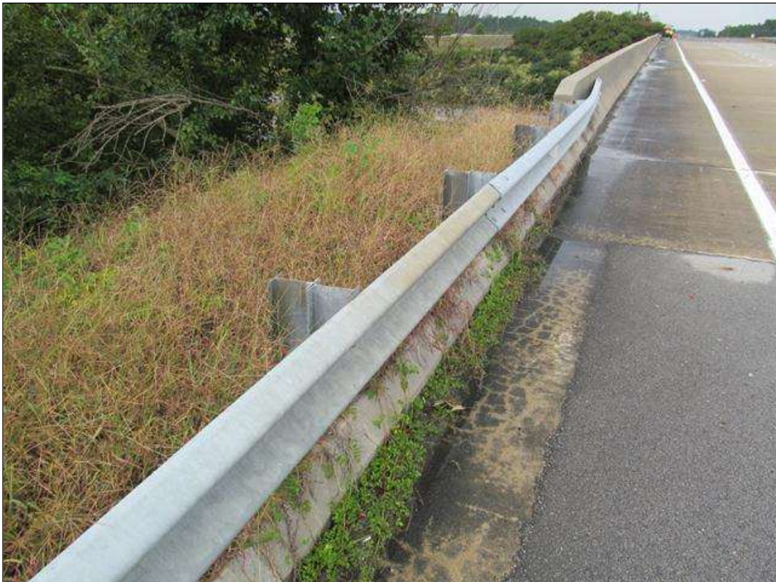
SE GUARDRAIL POST SPACINGS AT TRANSITION TO BRIDGE RAIL.
