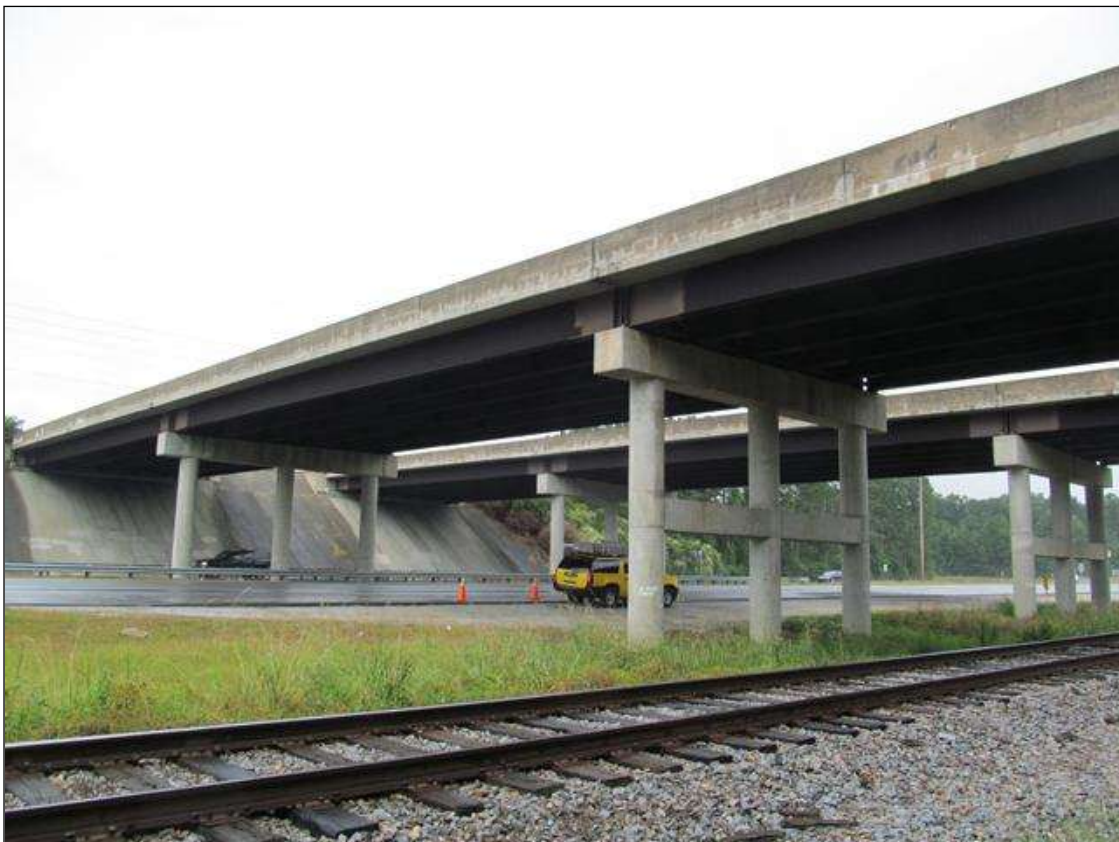
SOUTH SIDE, LOOKING WEST
