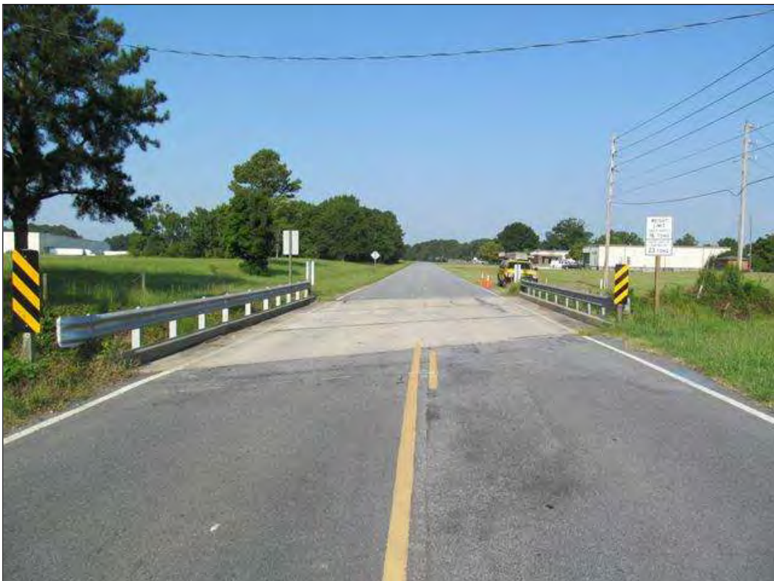
LOOKING WEST, SR 1591
