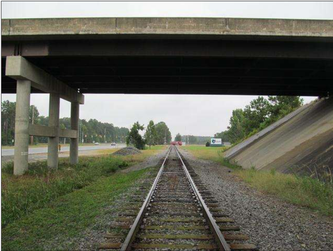
SPAN 3 CLEARANCE, LOOKING NORTH CSX RAILROAD.
