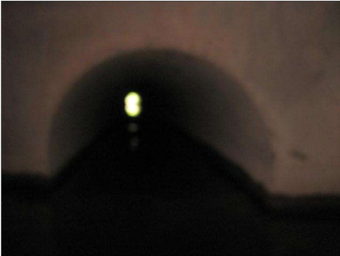
5' DIAMETER DRAINAGE PIPE, 530 FEET IN FROM SOUTH END, BARREL 3
