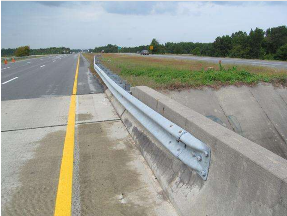
NW GUARDRAIL CONNECTION. (SW & SE CONNECTIONS SIMILAR)
