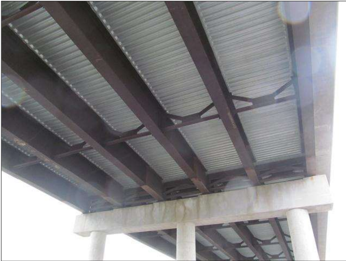
SPAN 1 UNDERSIDE. SPANS 1 & 3 SIMILAR
