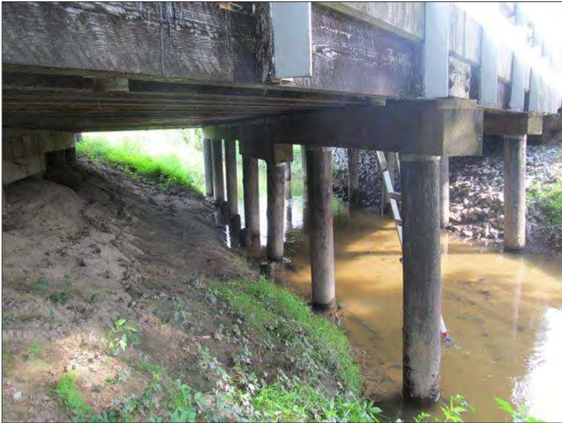
SPAN 1 SIDE OF BT.1. BT.2 SIMILAR.
