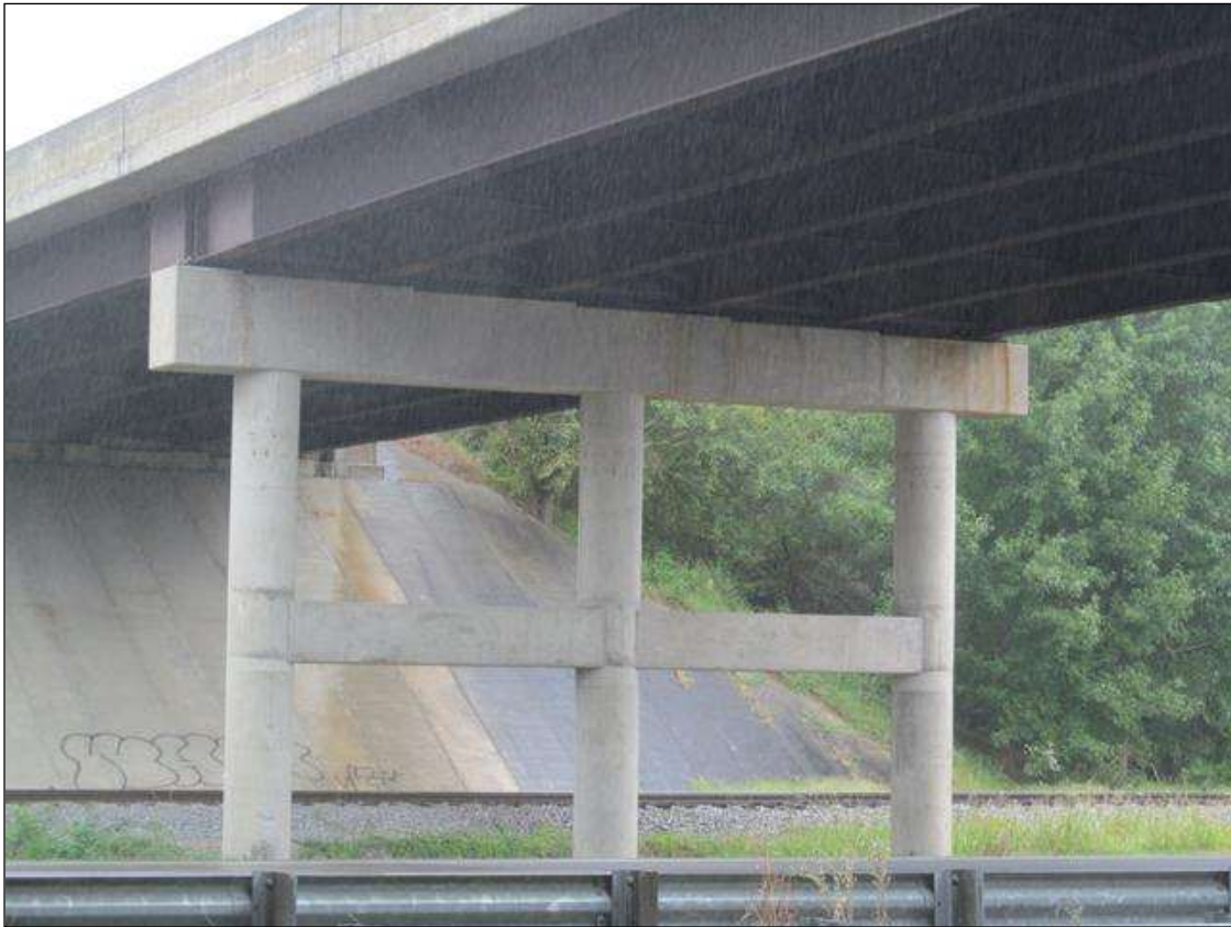
SPAN 2 SIDE OF BT 2
