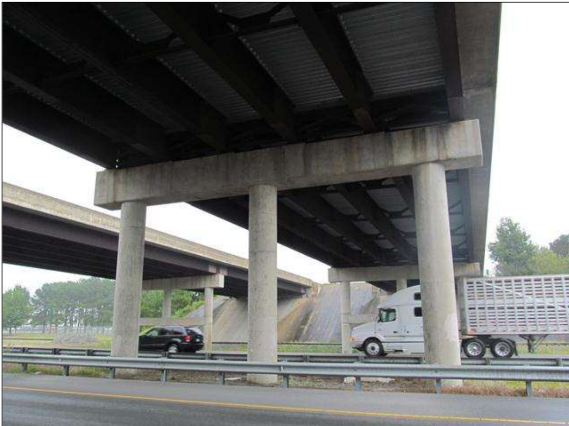
SPAN 1 SIDE OF BT 1
