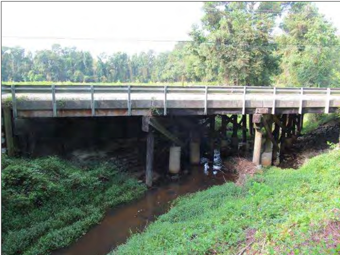
NORTH SIDE, LOOKING SOUTH
