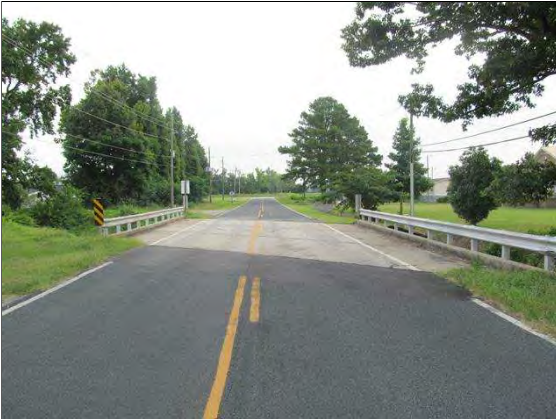
LOOKING NORTH, SR 1529.
