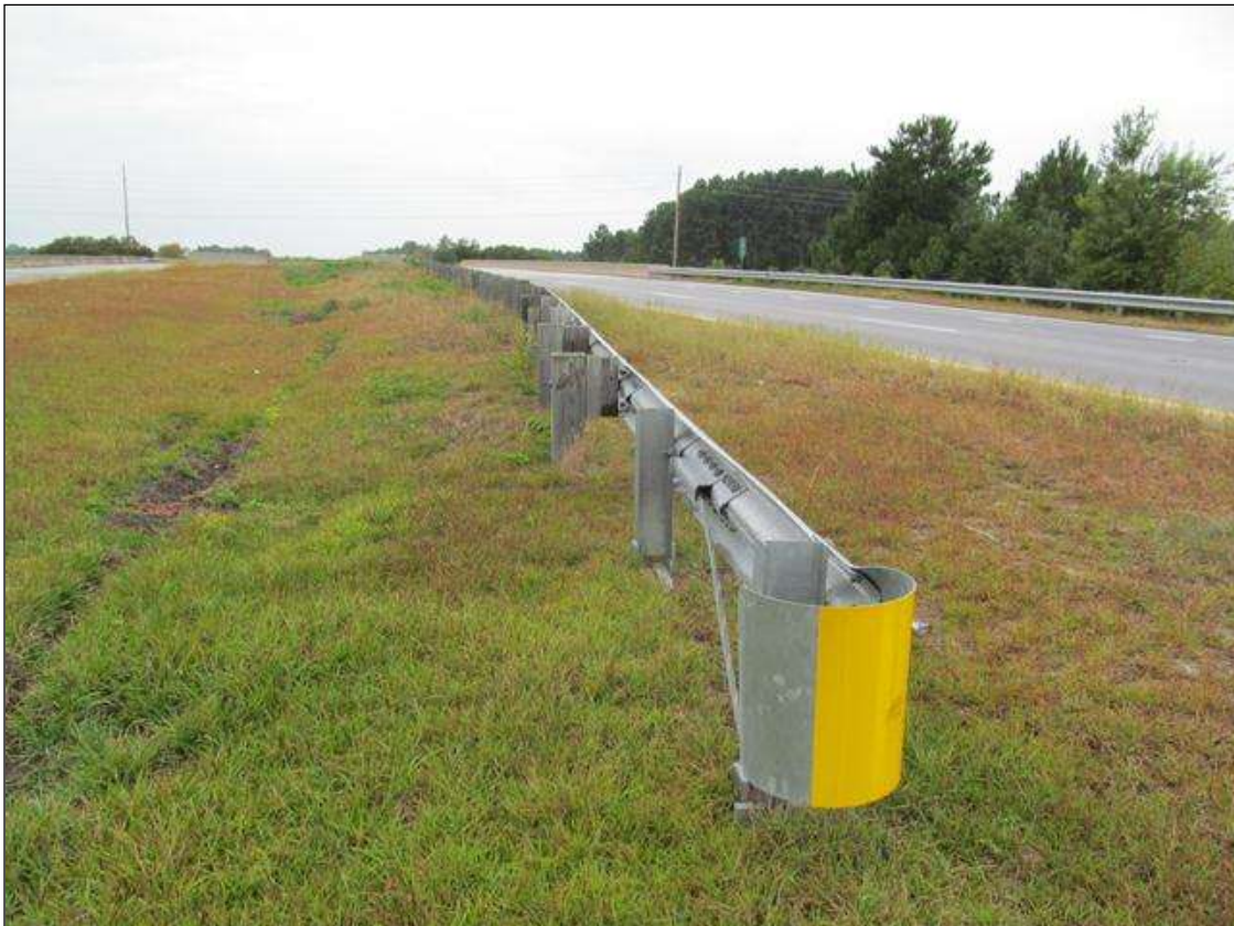
SE GUARDRAIL END. SIMILAR @ THE NE GUARDRAIL.
