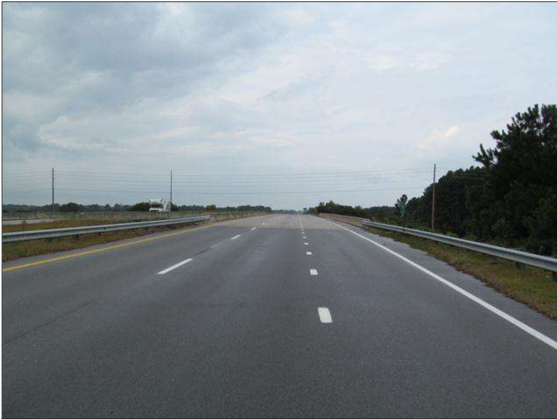
LOOKING WEST, US264 WEST BOUND LANES.
