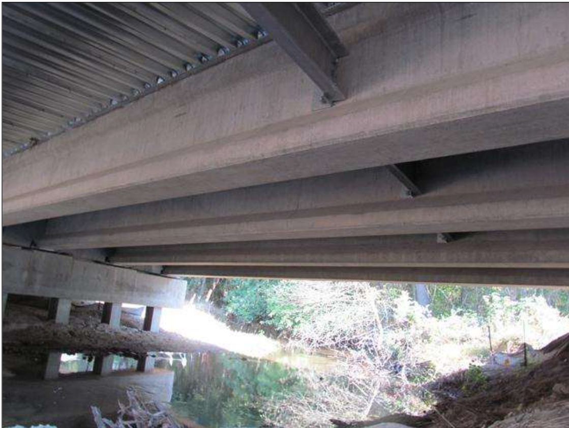
SPAN 2 UNDERSIDE. SPAN 1 SIMILAR.
