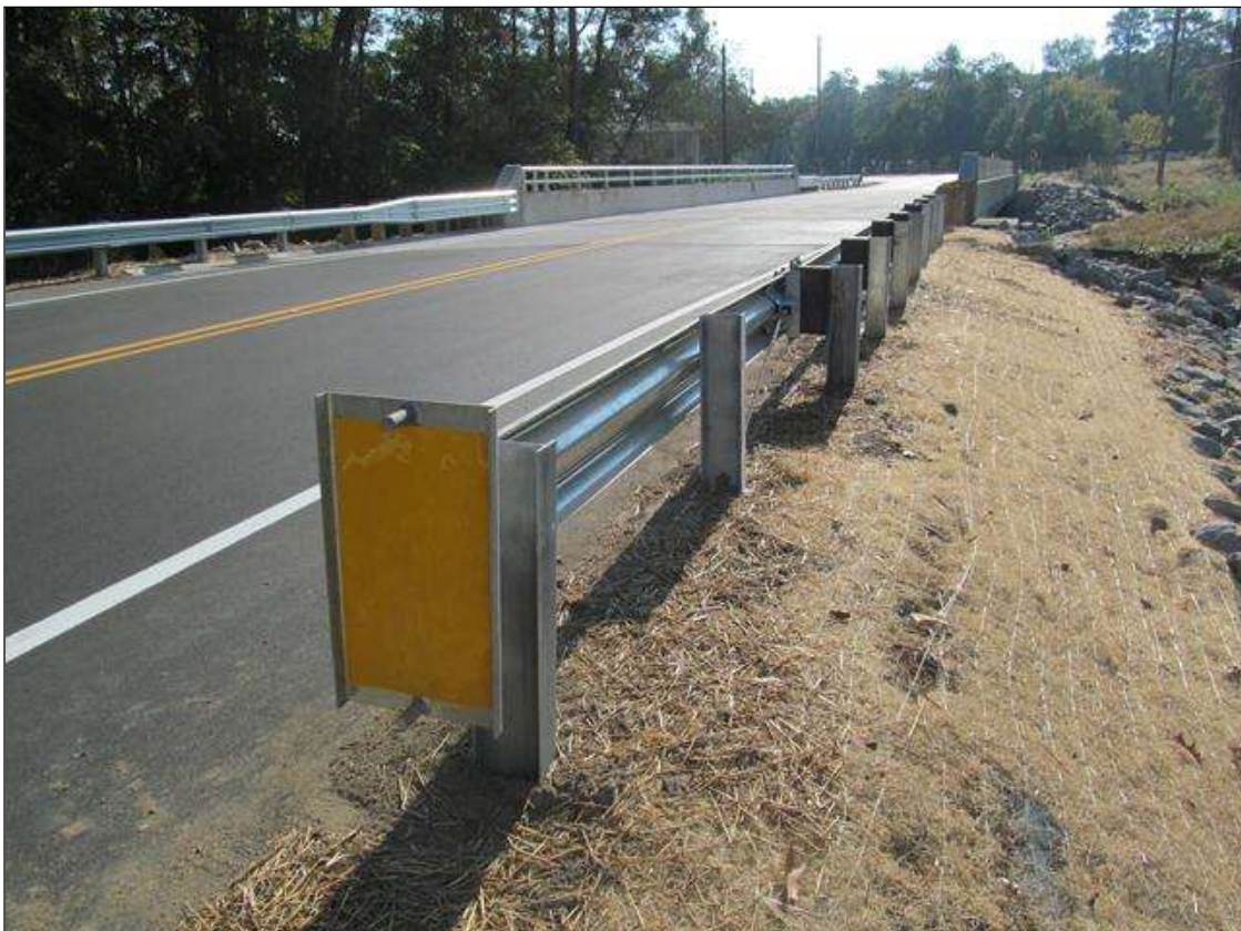
SW GUARDRAIL END. SIMILAR @ ALL GUARDRAILS.
