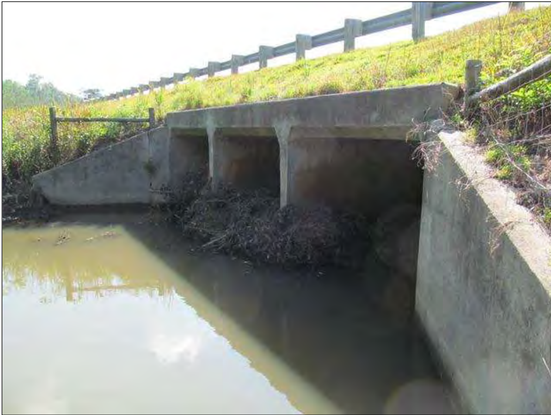
NORTH END, LOOKING EAST
