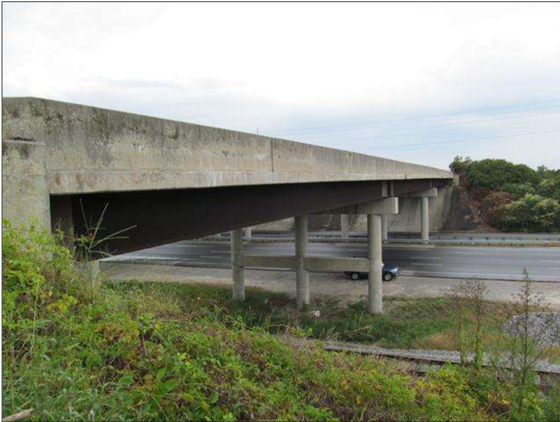
NORTH SIDE, LOOKING WEST.
