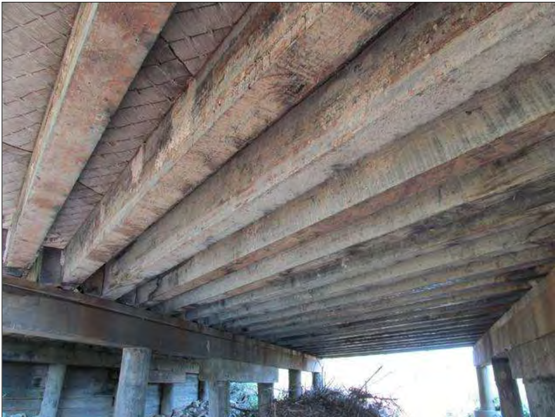
SPAN 2 UNDERSIDE. (SPANS 1 & 3 SIMILAR)
