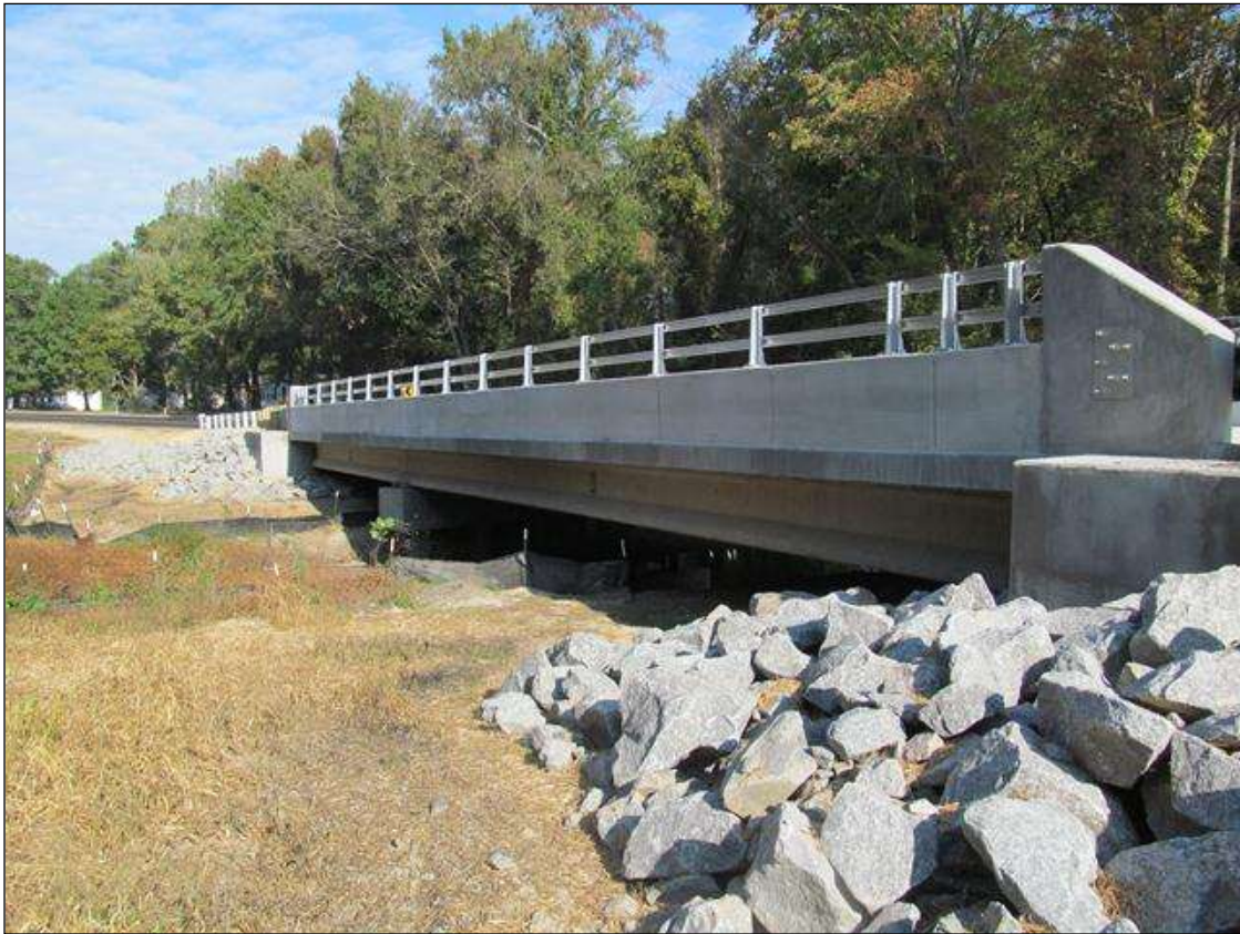
SOUTH SIDE, LOOKING WEST.
