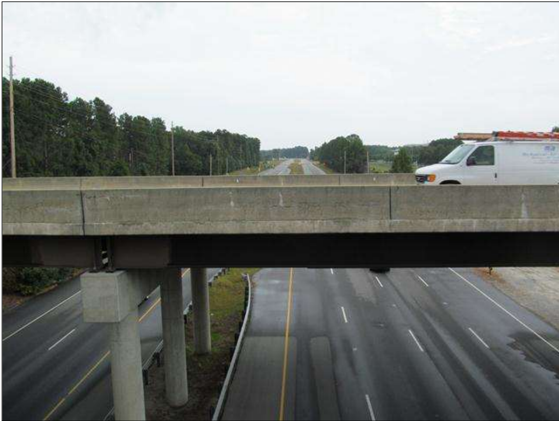
LOOKING NORTH, US13/NC11/NC903
