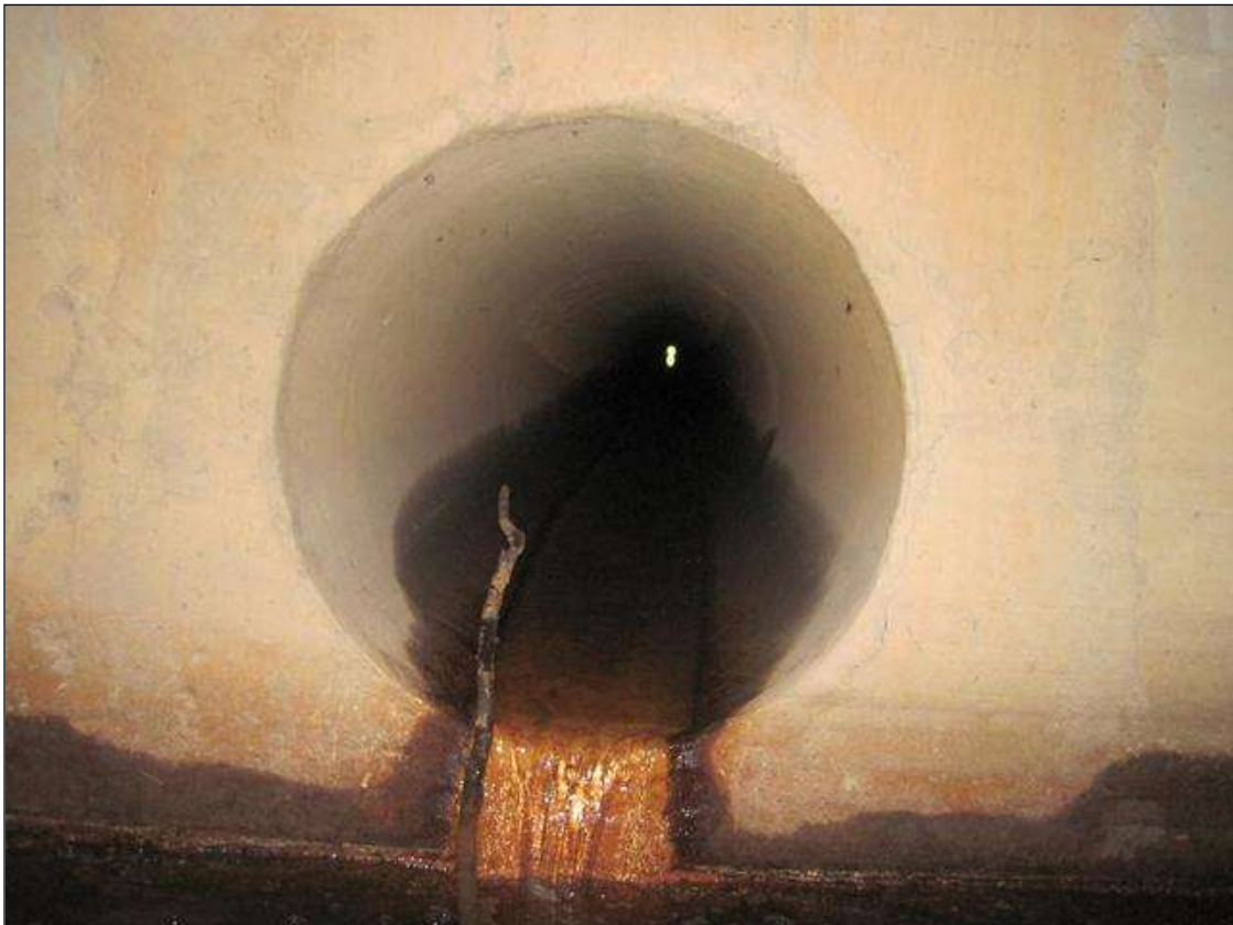
DRAINAGE PIPE, 300 FEET FROM SOUTH END. BARREL 1
