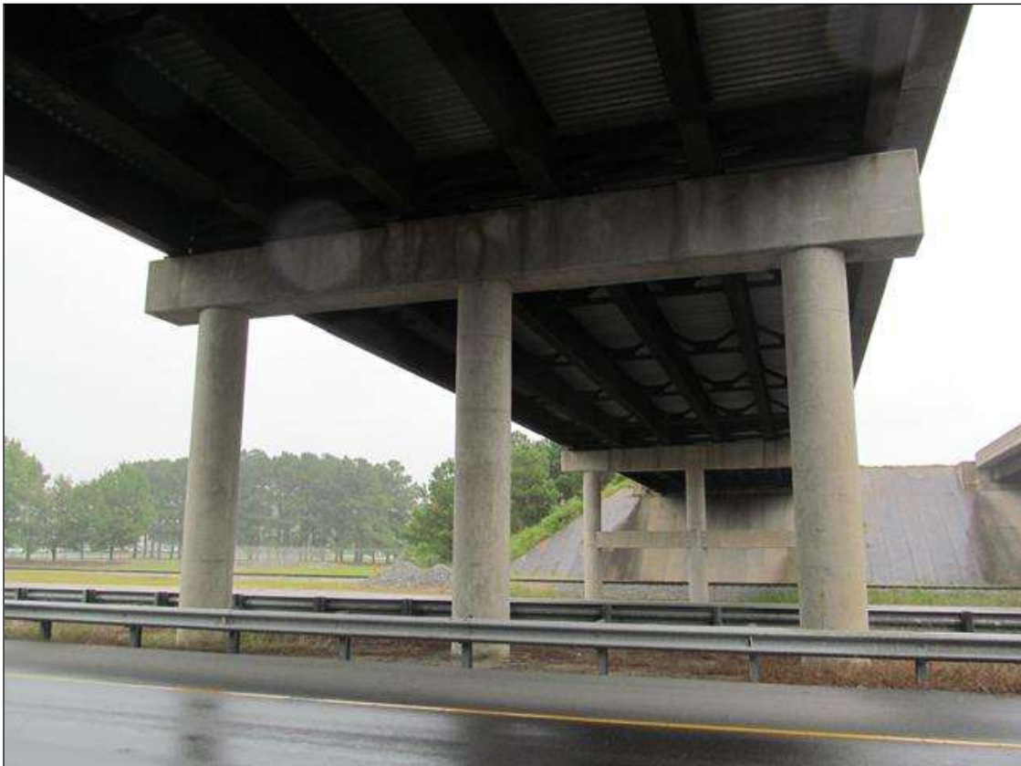
SPAN 1 SIDE OF BT.1
