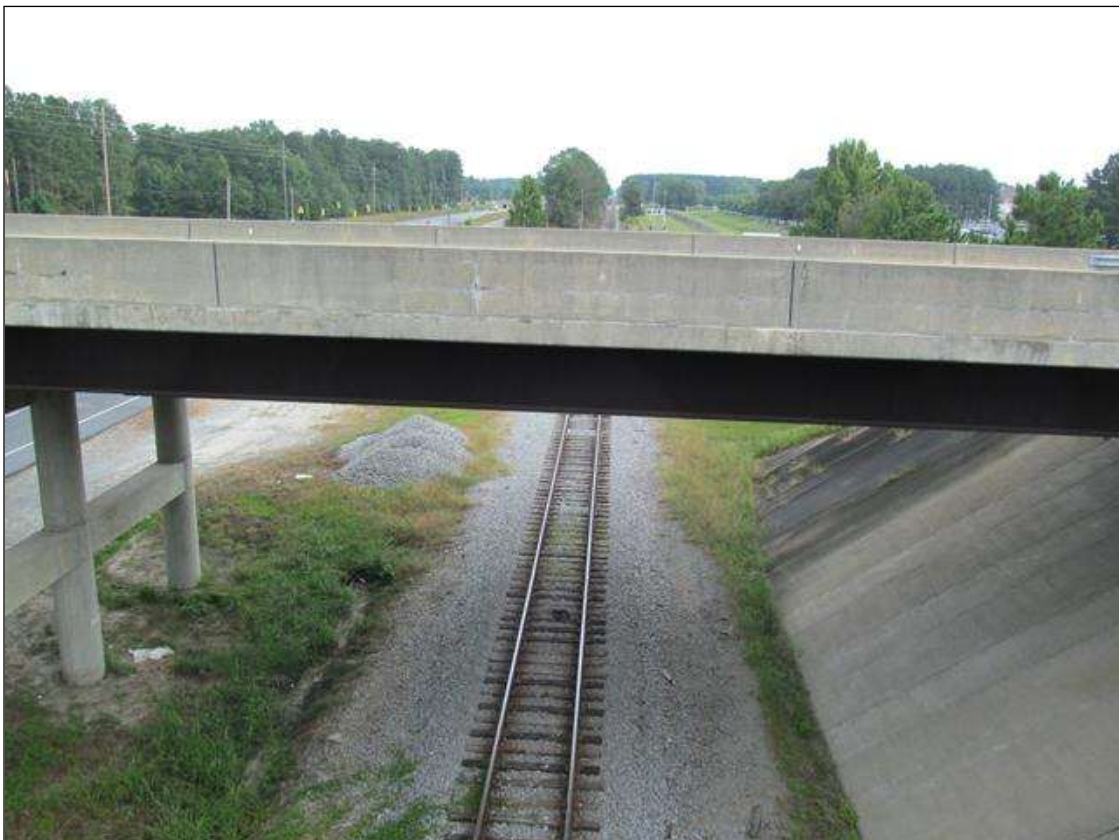
LOOKING NORTH, CSX RR
