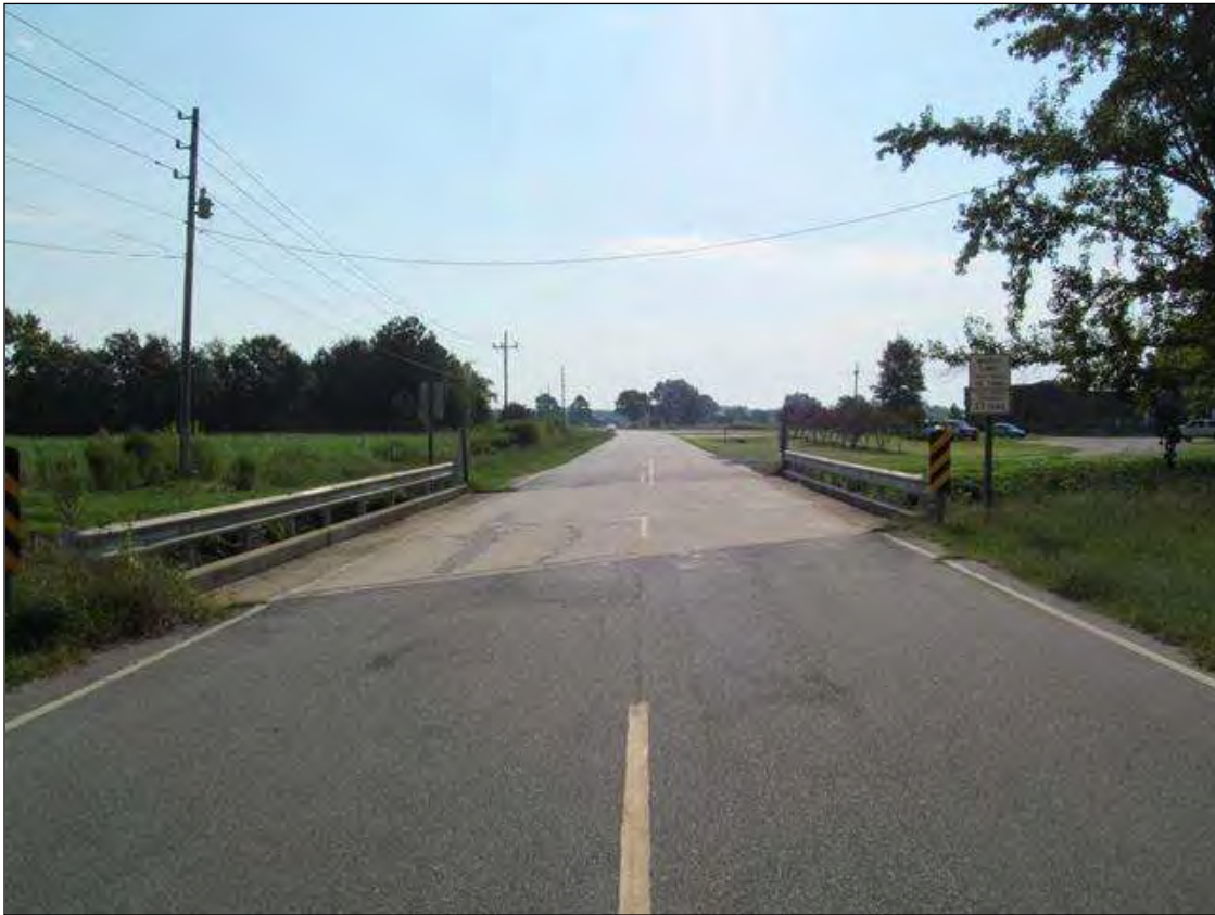
LOOKING EAST, SR 1591
