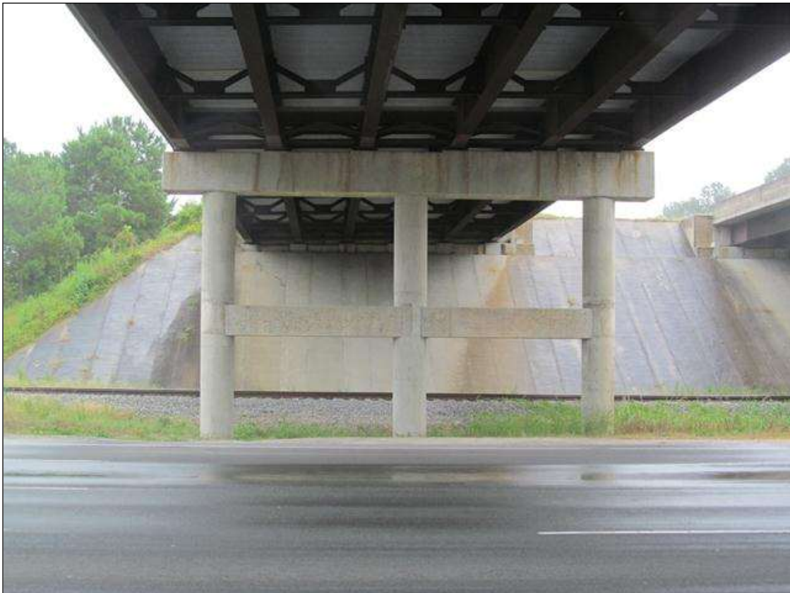
SPAN 2 SIDE OF BT.2
