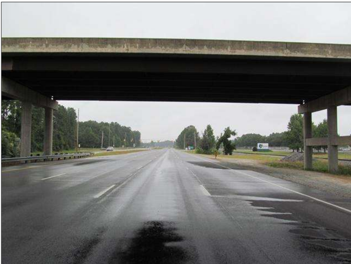
SPAN 2 CLEARANCES, LOOKING NORTH US13/NC11/NC903.
