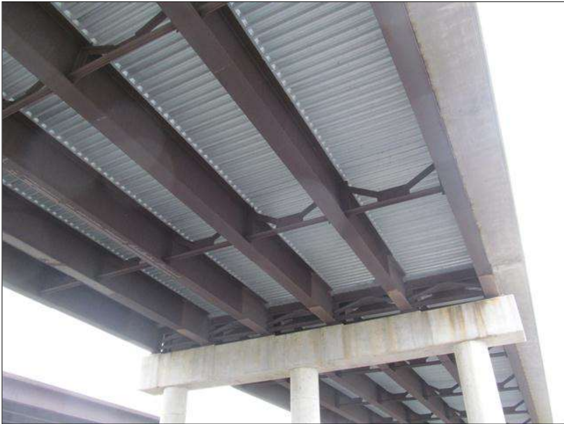
SPAN 1 UNDERSIDE. (ALL SPANS SIMILAR)
