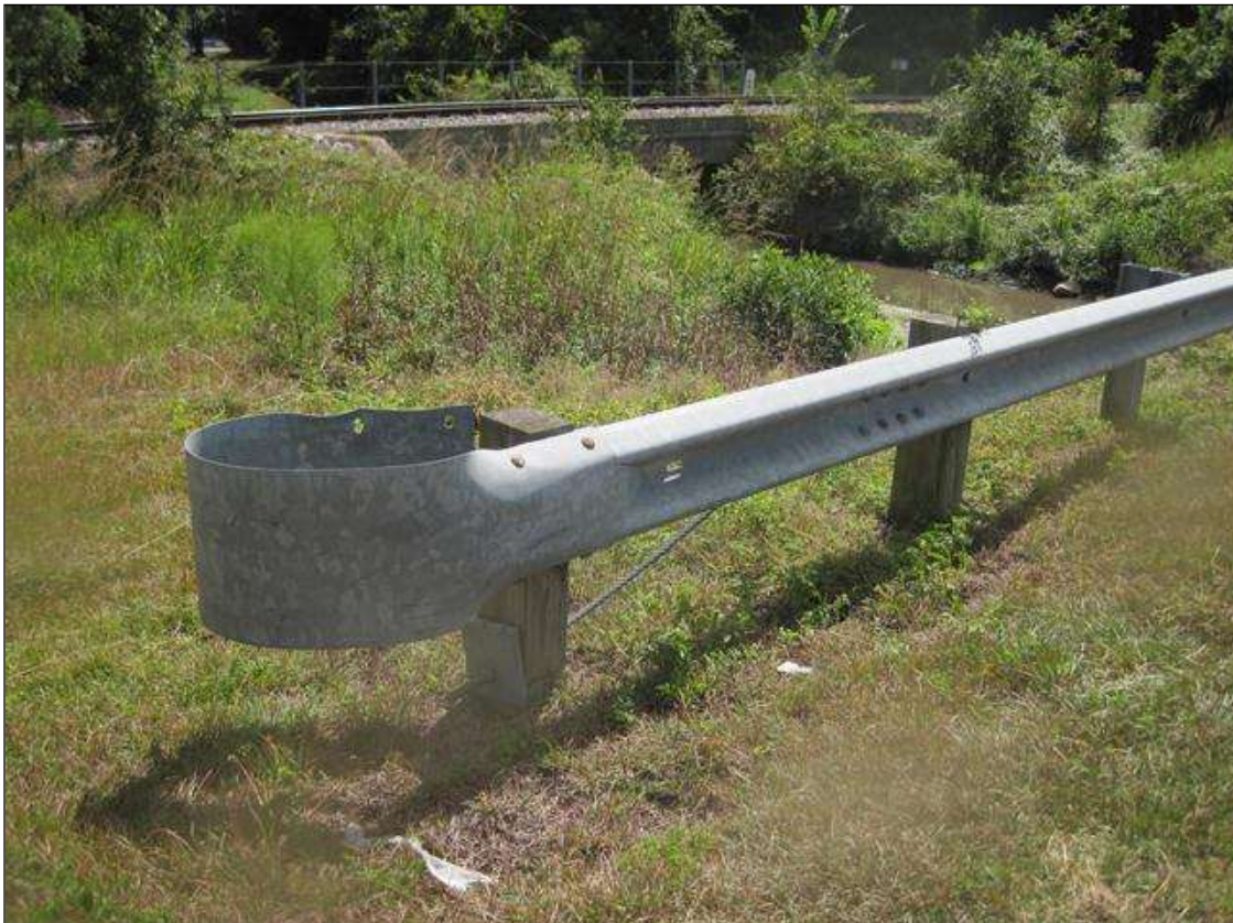
GUARD RAIL END
