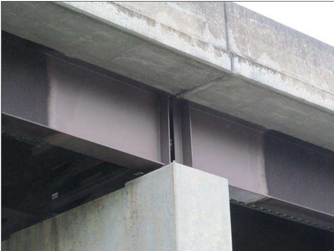
WEATHERING STEEL WITH COATED ENDS.
