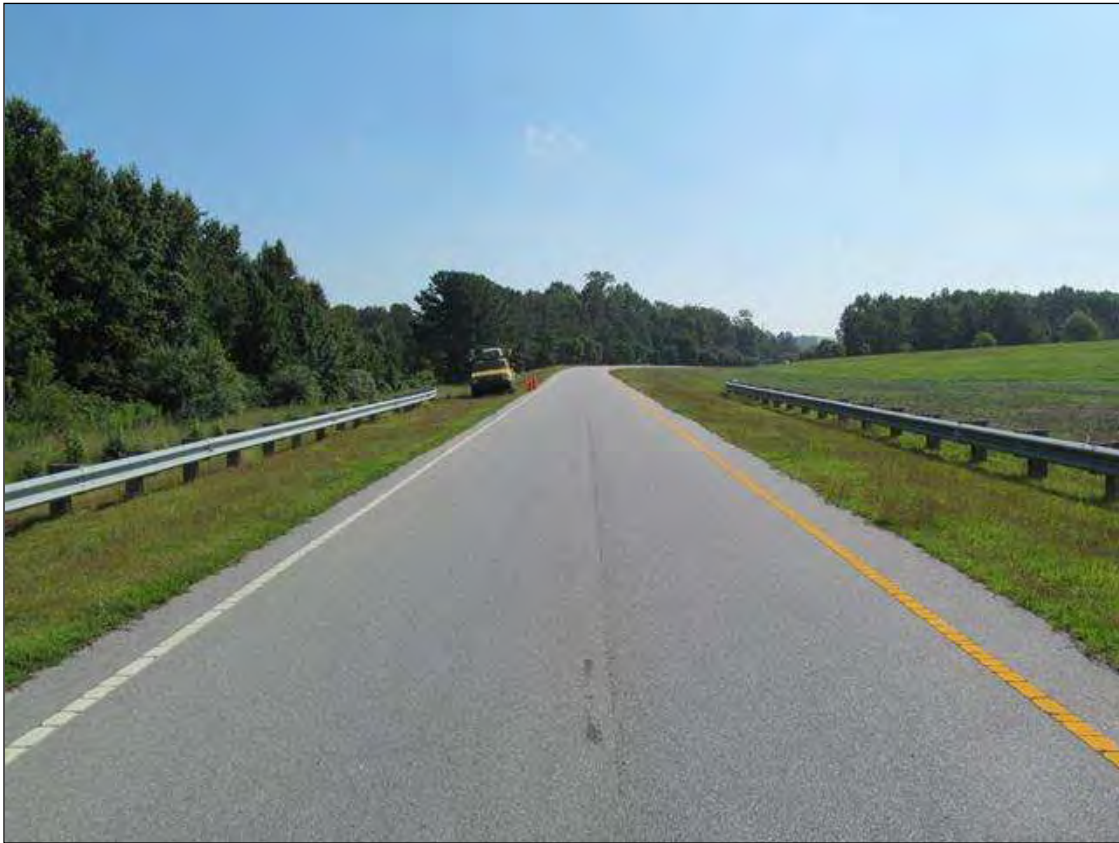
LOOKING EAST, RAMP TO US 264 W. BOUND.
