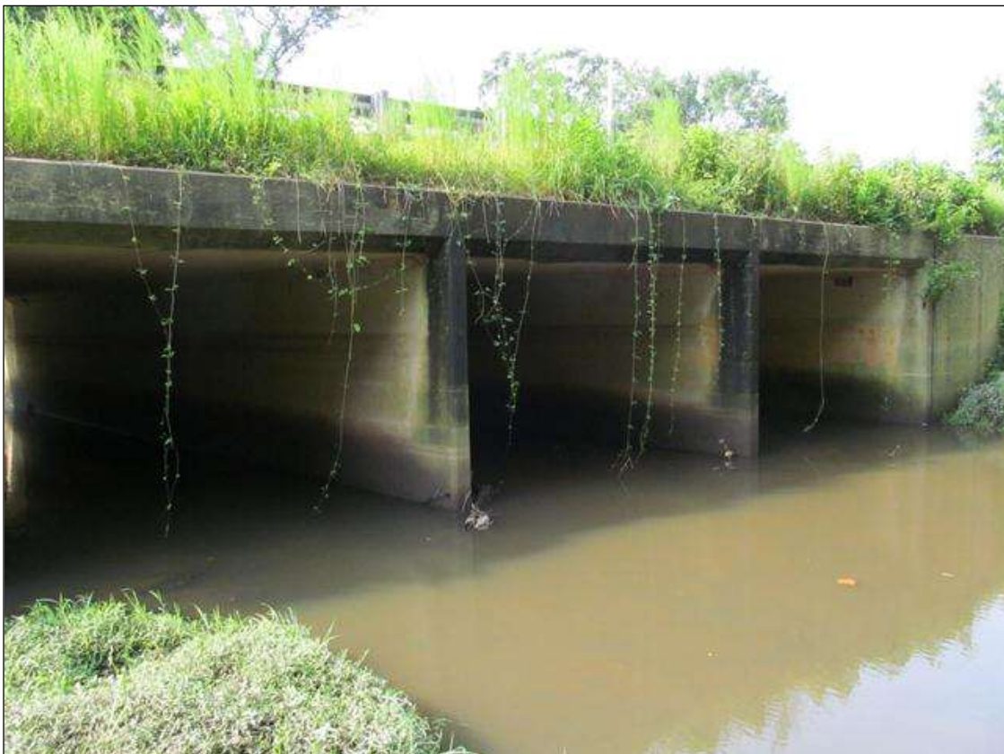
NORTH END, LOOKING WEST.
