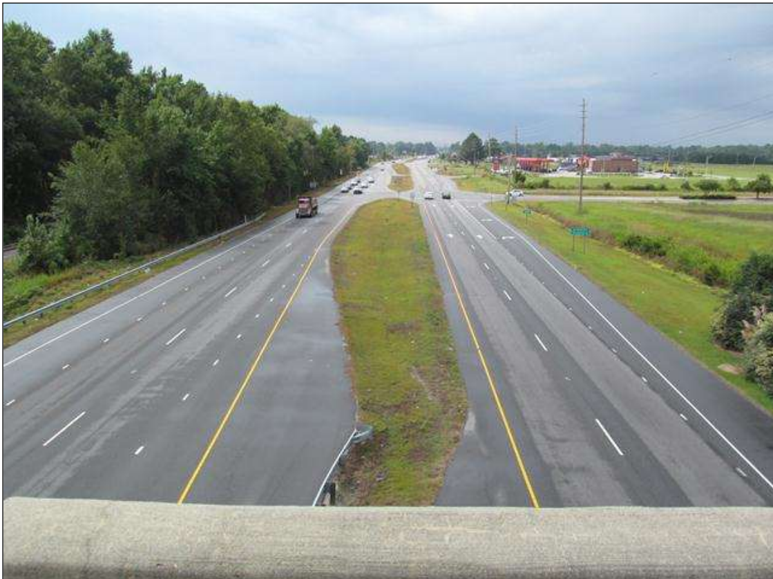
LOOKING SOUTH, US13/NC11/NC903
