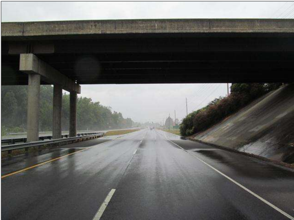
SPAN 1 UNDERCLEARANCE, LOOKING SOUTH, US 13/NC11/NC903 SB LANES TOWARDS GREENVILLE.
