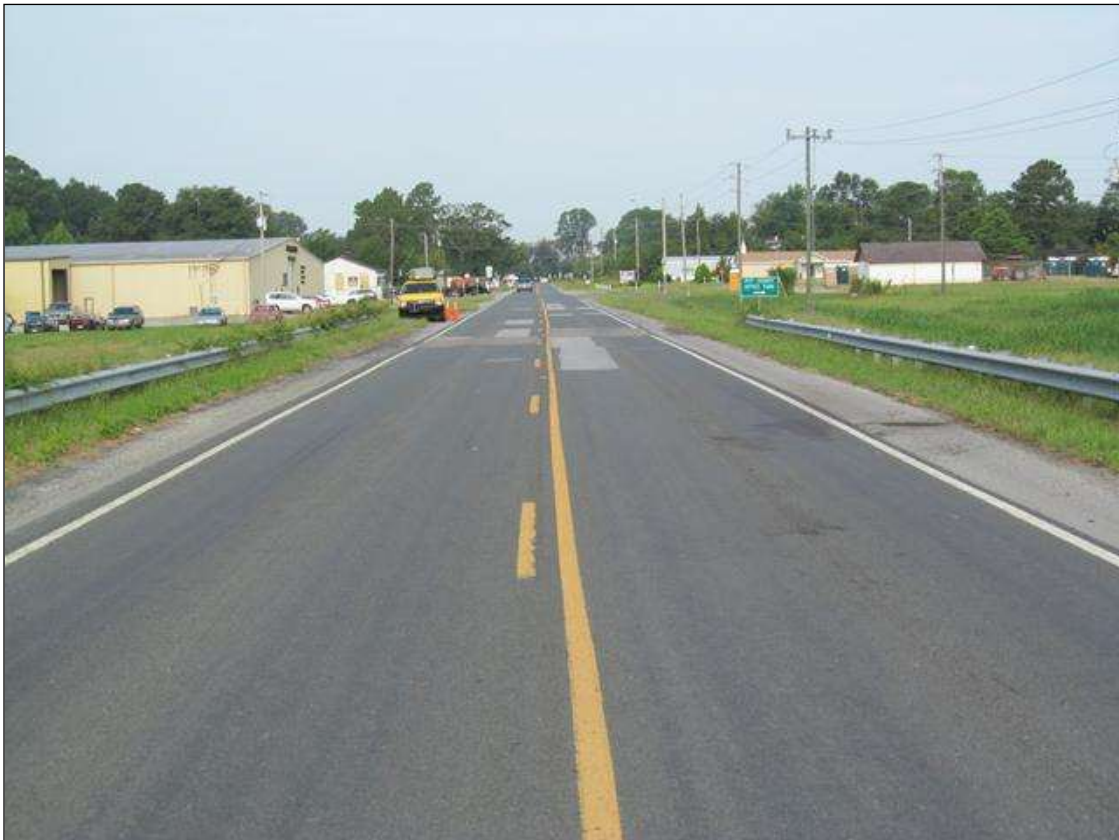
LOOKING WEST, SR1530.
