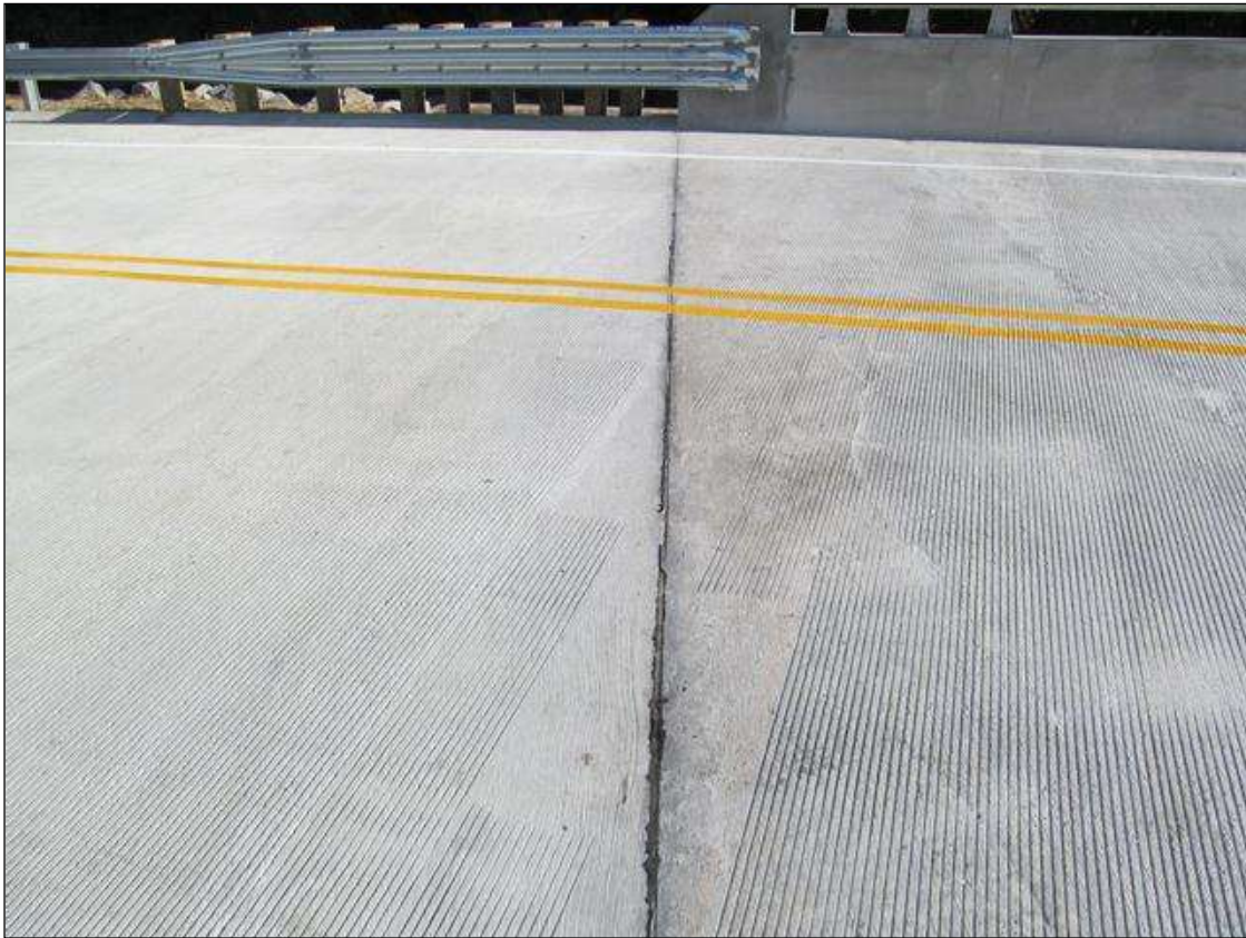
CONSTRUCTION JOINT @ EBT.1. SIMILAR @ EBT.2.
