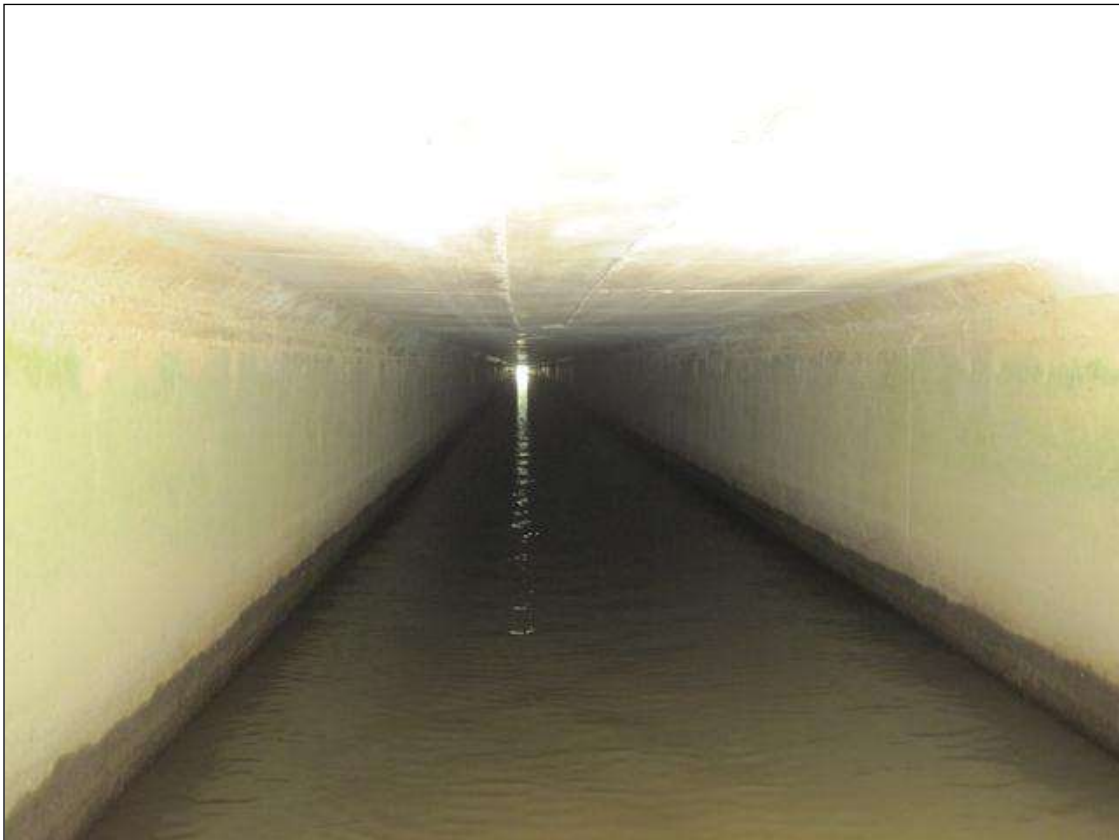
LOOKING NORTH THROUGH BARREL 2
