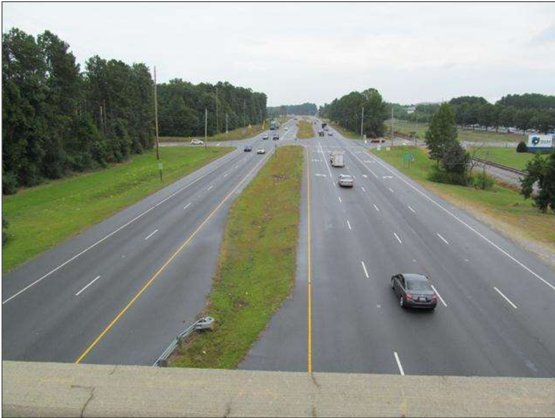
LOOKING NORTH, US13/NC11/NC903.
