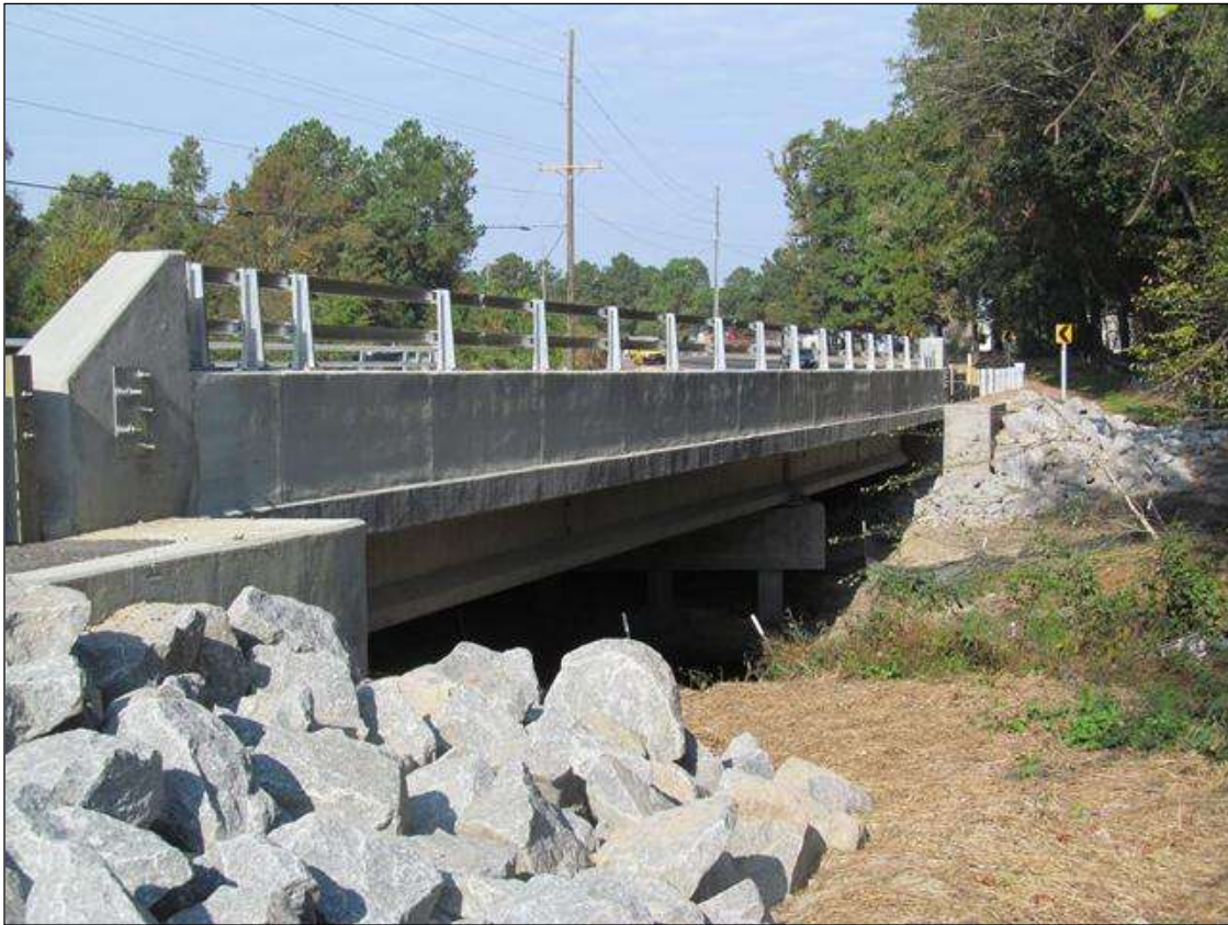
NORTH SIDE, LOOKING WEST.
