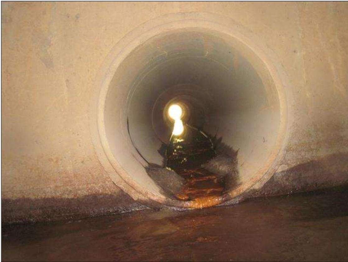
DRAIN PIPE, 200 FEET FROM NORTH END. BARREL 1
