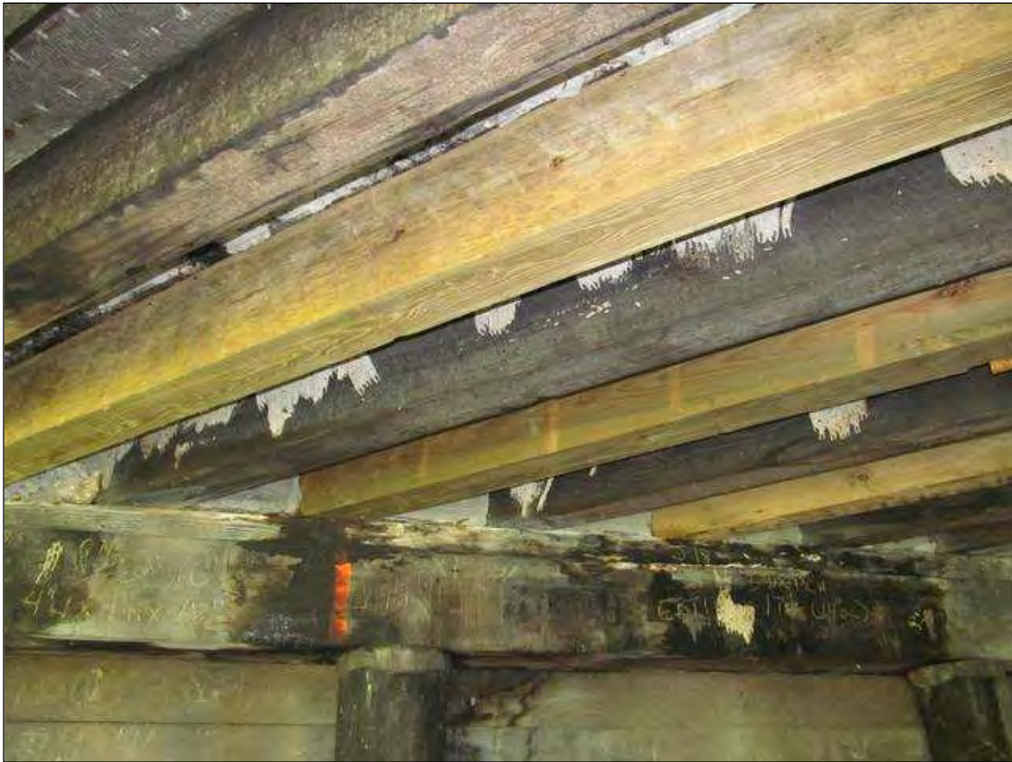
J-18 & 22 IN SPAN 1 HAVE BEEN REPLACED PER PM ISSUED LAST CYCLE.
