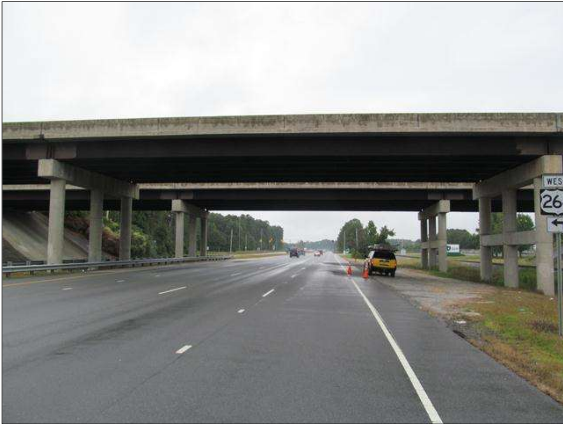
SPAN 2 UNDERCLEARANCE, LOOKING NORTH, US 13/NC11/NC903 NB LANES TOWARDS BETHEL
