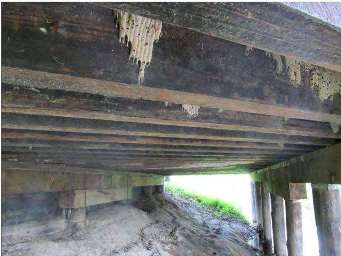
SPAN 1 UNDERSIDE. SIMILAR IN ALL SPANS.
