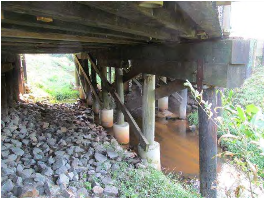
SPAN 1 SIDE OF BT 1
