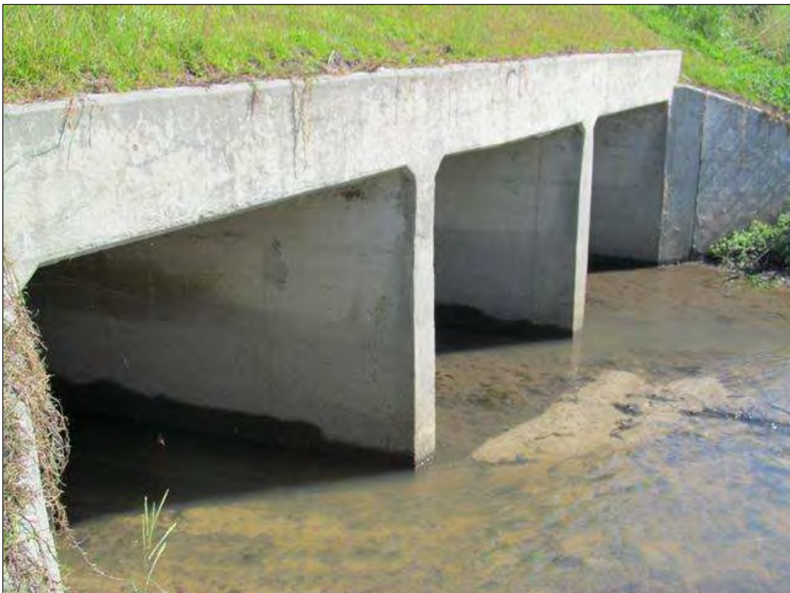
SOUTH END, LOOKING EAST
