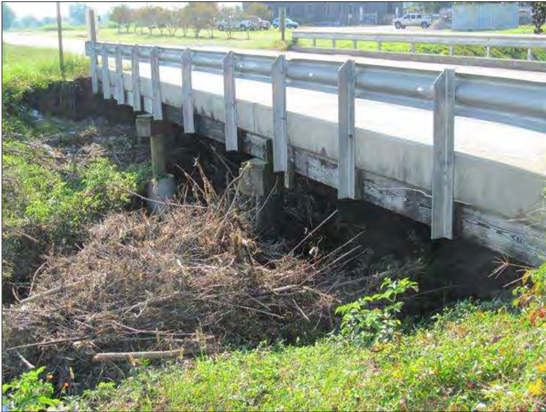
NORTH SIDE, LOOKING EAST
