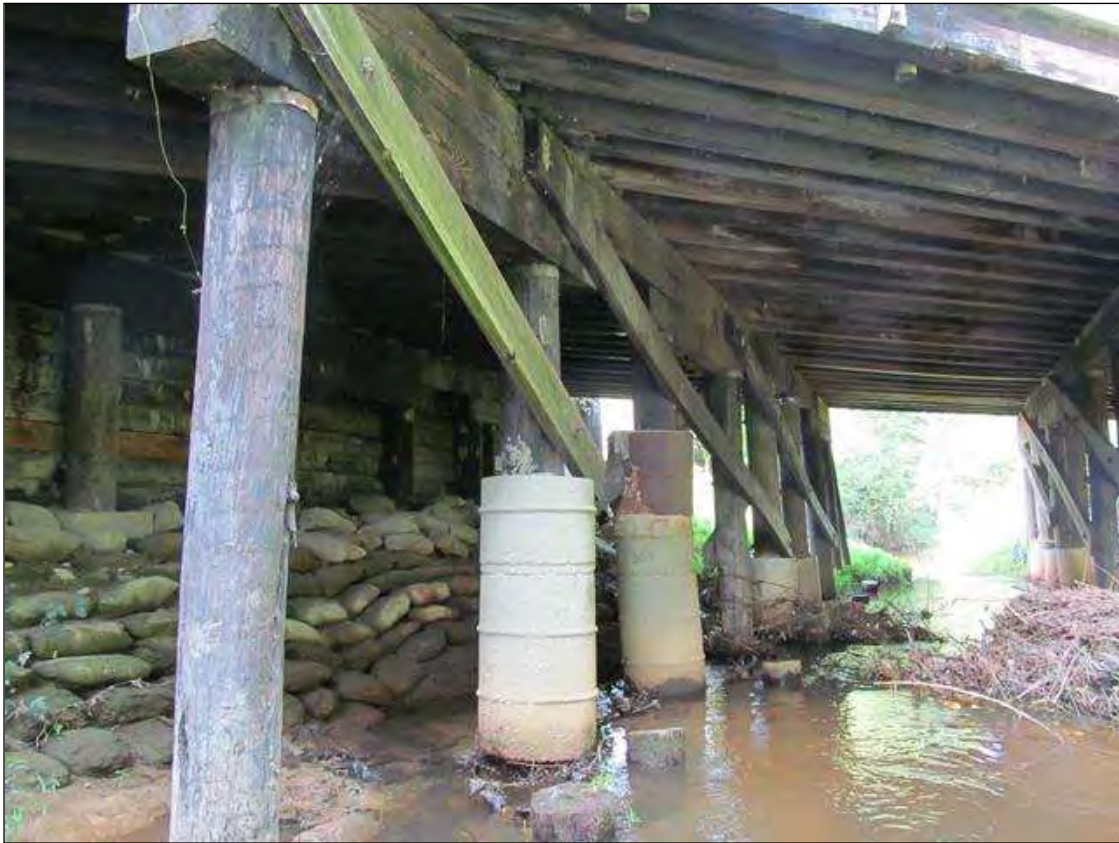
SPAN 2 SIDE OF BENT 2
