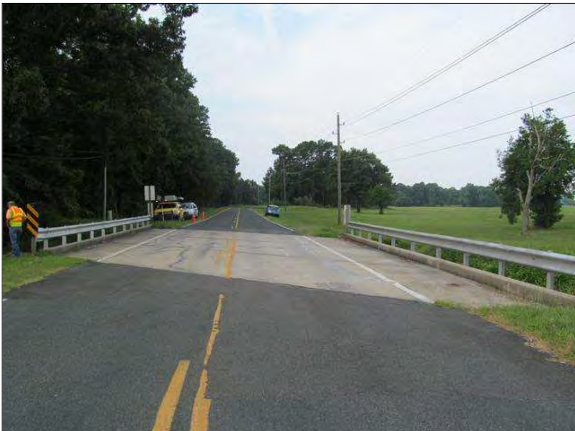
LOOKING SOUTH, SR 1529.
