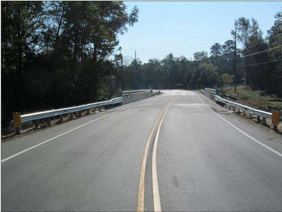
LOOKING EAST, SR 1401.
