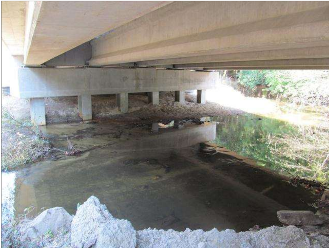
SPAN 2 SIDE OF BT.1.
