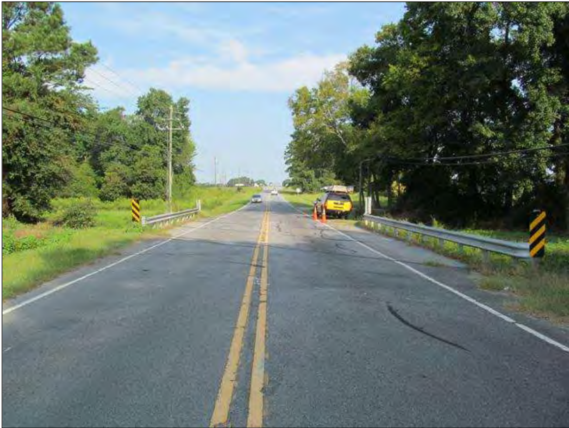
LOOKING WEST, NC 33
