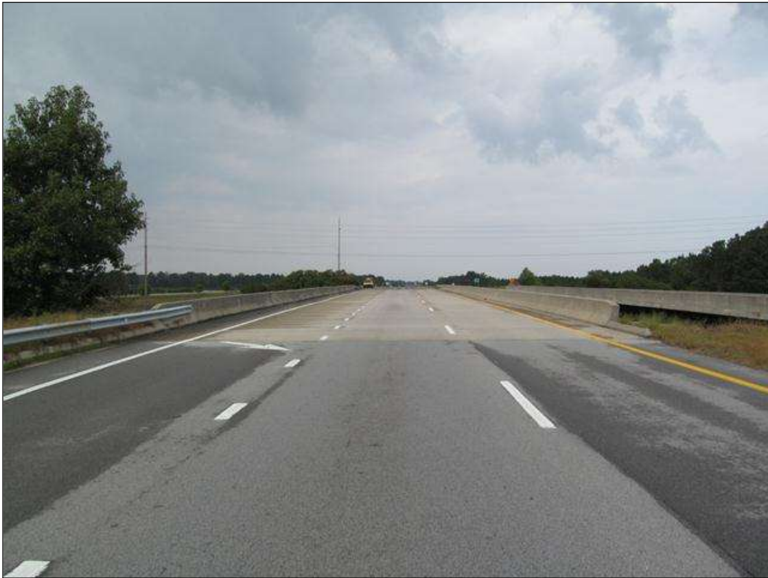
LOOKING WEST, US 264 BYP, EB LANES
