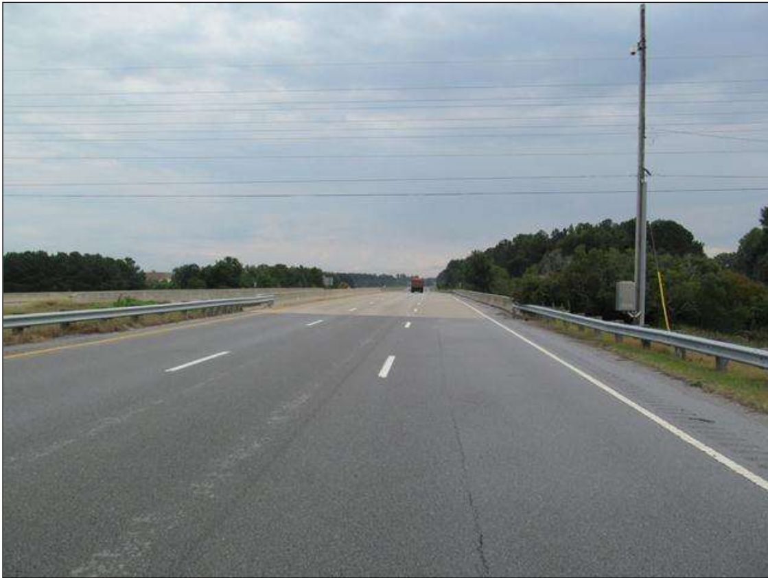
LOOKING EAST, US 264 BYP, EB LANES
