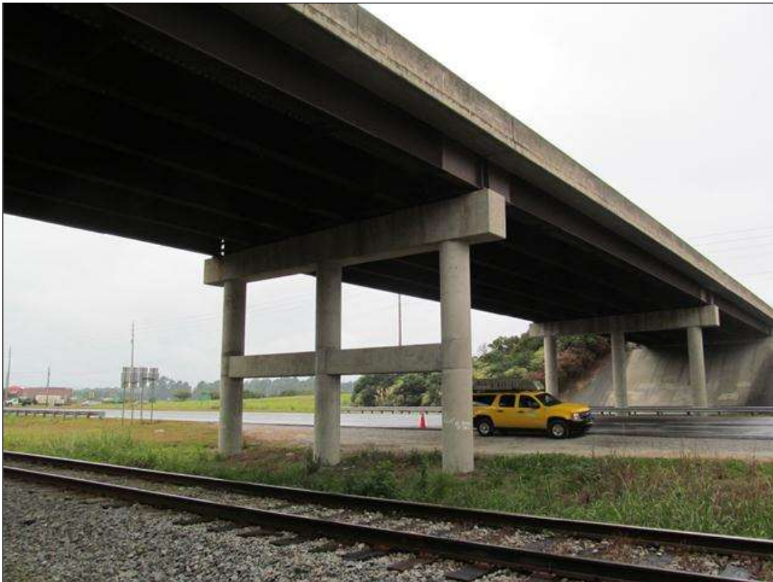
NORTH SIDE, LOOKING WEST
