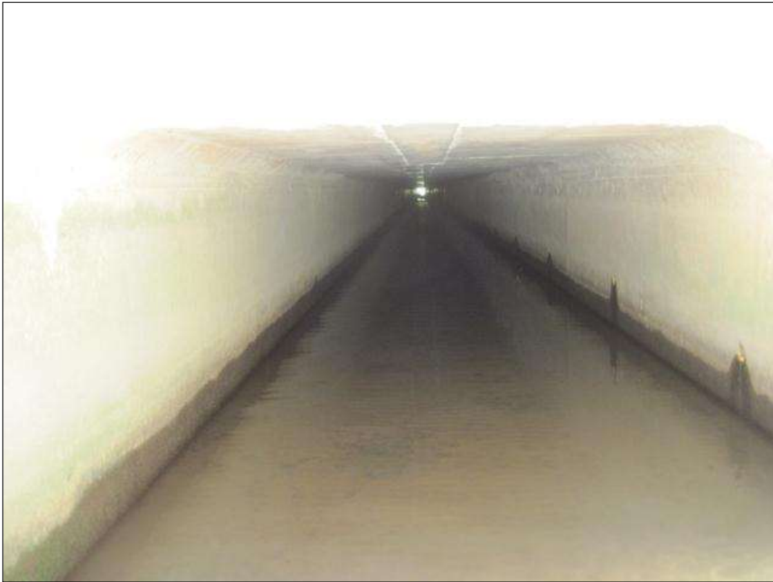
LOOKING NORTH THROUGH BARREL 3
