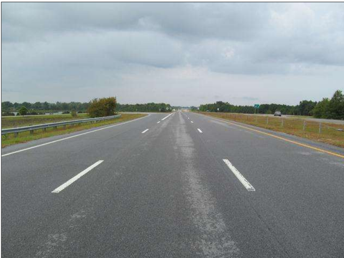
LOOKING WEST AT US 264EB LANES & ON RAMP FROM US13/NC11/NC903 SB
