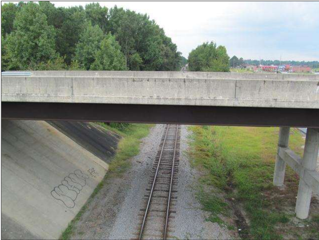
LOOKING SOUTH, CSX RAILROAD
