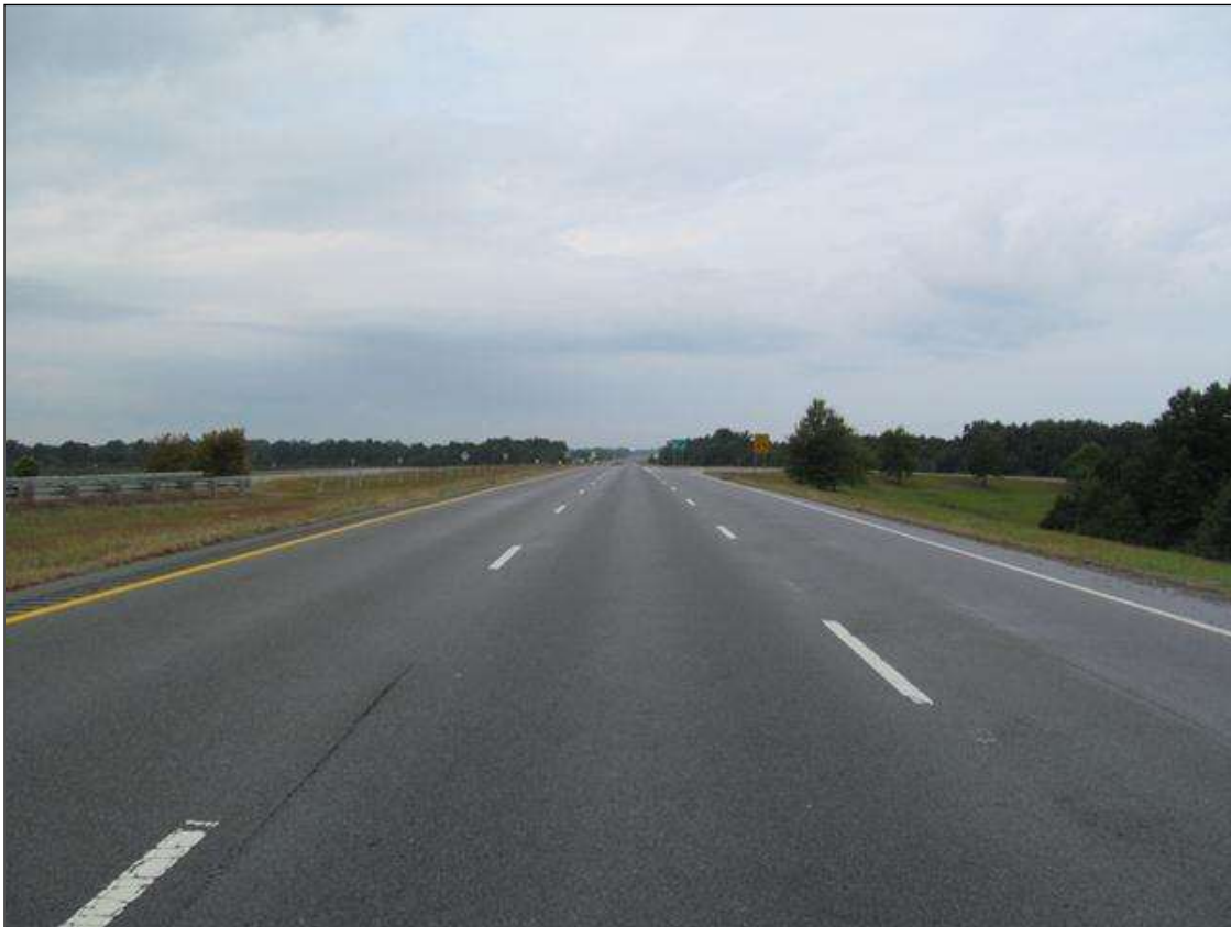
LOOKING WEST @ THE OFF RAMP TO US13/NC11/NC903.
