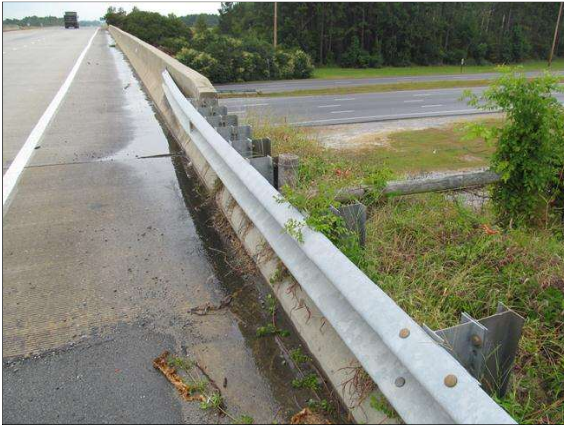
NE GUARDRAIL POST SPACINGS @ THE TRANSITION. SIMILAR @ THE SE GUARDRAIL.
