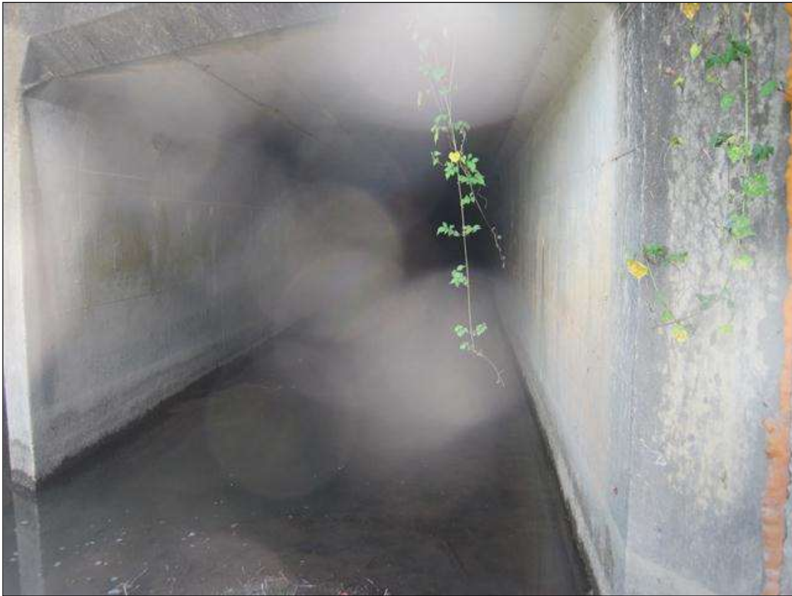
LOOKING NORTH THROUGH BARREL 1
