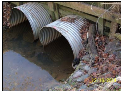
Picture 3-2. Sterling Trace Drive –Upstream Face
