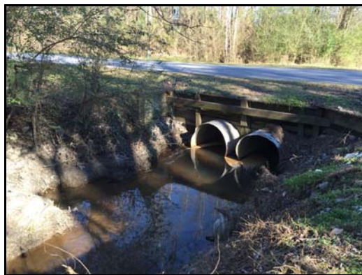
Picture 4-1. Sterling Trace Drive – Existing CMPs
