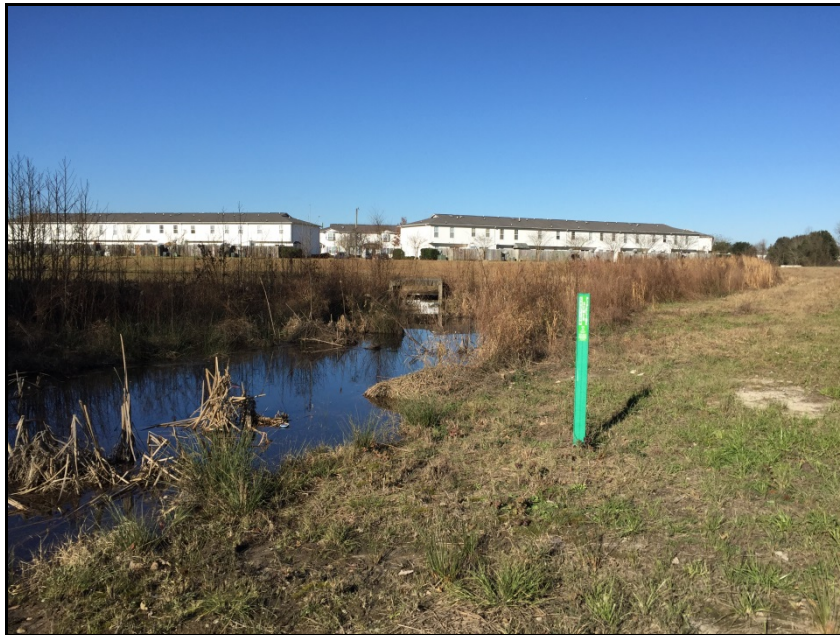
Picture 5-13. Proposed Location for Sterling Pointe Apartments Wet Pond Retrofit
