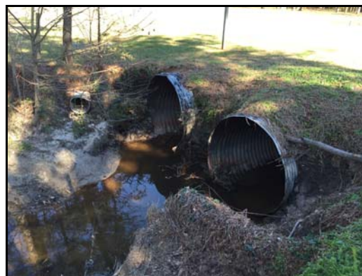
Picture 4-4. Frog Level Road – Existing CMPs
