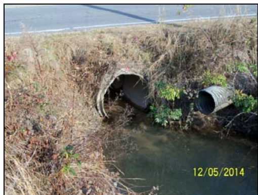
Picture 4-2. Thomas Langston Drive – Existing RCP
