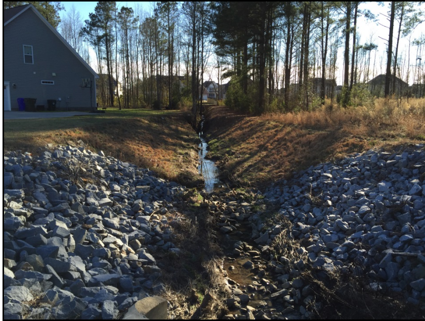
Picture 5-11. Proposed Location for South Bend Regenerative Stormwater Conveyance
