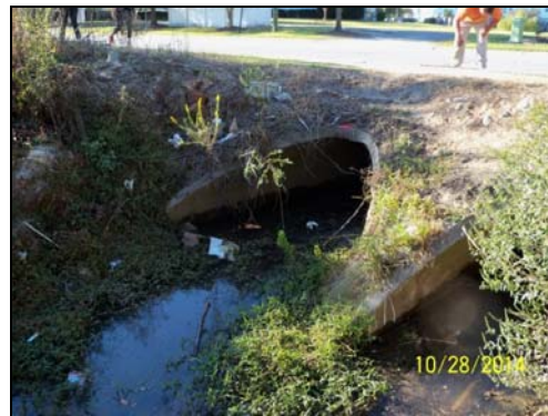
Picture 4-3. Sterling Pointe Drive – Existing RCPs
