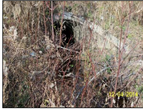
Picture 3-4. Belfair Drive – Downstream Face
