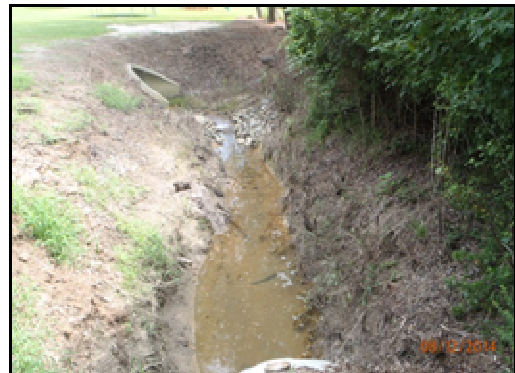
Picture 5-1: Outfall at top of project
