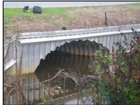
Picture 3-6. Corey Road Culvert – Upstream Face
