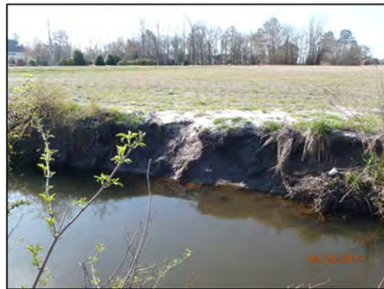
Picture 5-4. Erosion and lack of riparian buffer downstream of Corey Road
