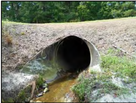
Picture 4-1. East Baywood Lane Culvert – Upstream Face
