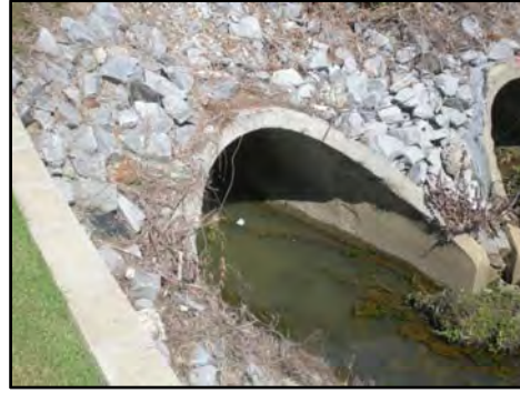
Picture 3-10. East Tower Road –U/S Culvert – Upstream Face
