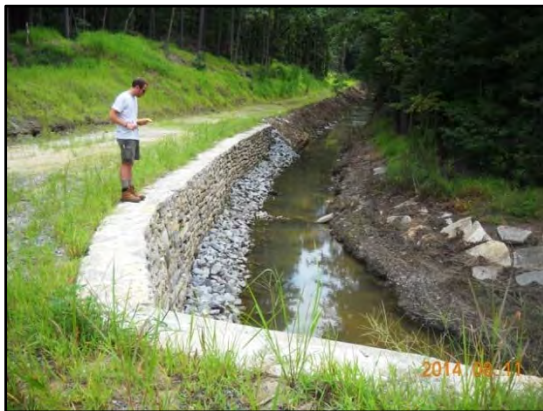
Picture 5-10. Armored 90-degree bend
