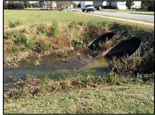
Picture 4-2. Trafalgar Drive – South Culverts
