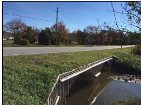
Picture 4-3. Corey Road CMP arches
