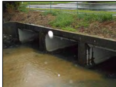
Picture 3-8. Coleman Drive Culvert – Downstream Face
