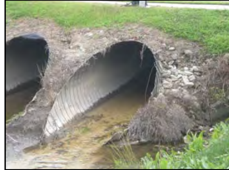
Picture 3-4. Trafalgar Drive – South Culvert – Downstream Face
