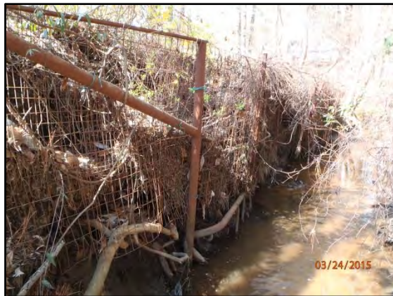
Picture 5-13. Vertical stream bank behind property at 3307 Evans Street
