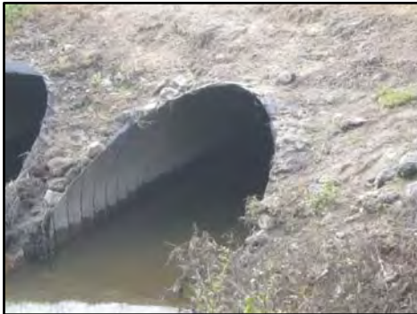
Picture 3-5. Trafalgar Drive – North Culvert – Downstream Face
