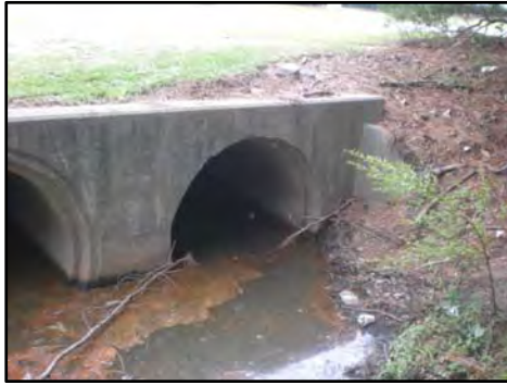
Picture 3-9. County Home Road Culvert – Upstream Face
