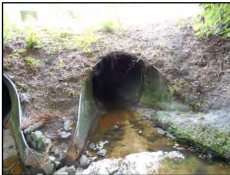
Picture 3-1. East Baywood Lane Culvert – Upstream Face
