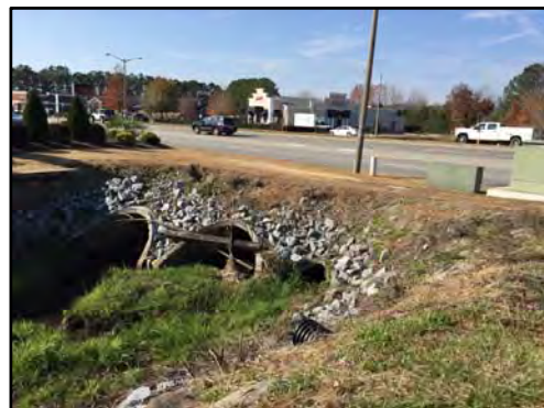
Picture 4-5. East Fire Tower Road –U/S RCPs
