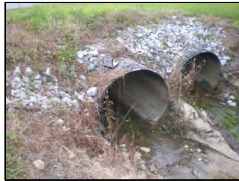
Picture 3-12. Tower Place Culvert – Downstream Face
