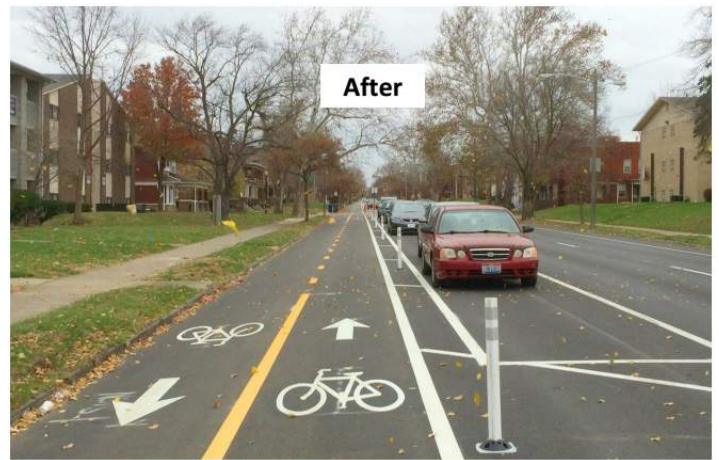
Street Resurfacing and Restriping
