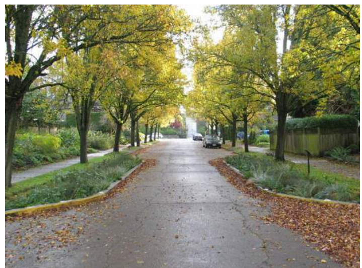
Bioretention Traffic Calming
