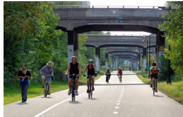
Midtown Greenway in Minneapolis, Minnesota utilizes an existing rail bed to connect population and employment centers.
