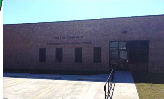
EMERGENCY OPERATIONS CENTER
