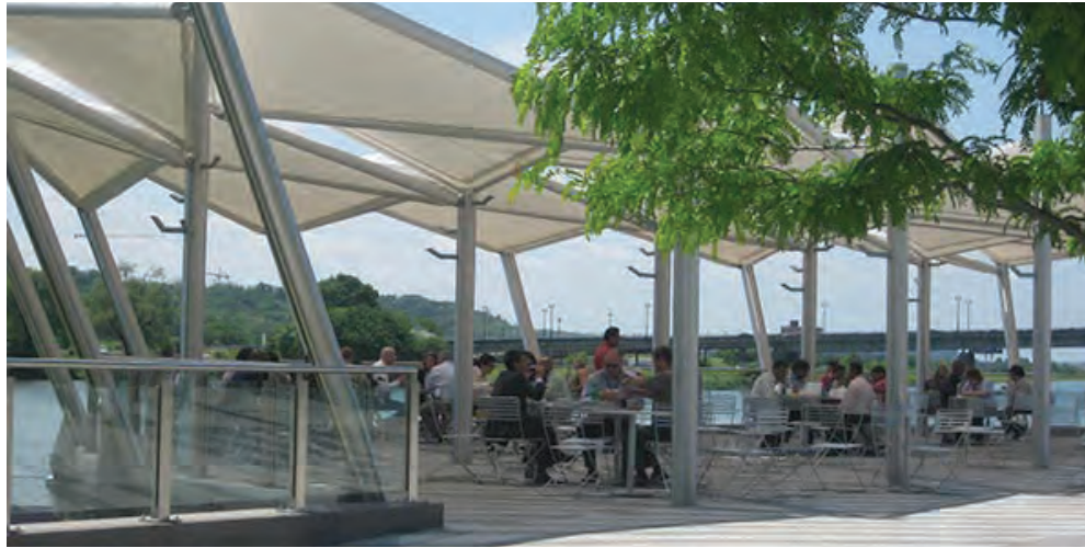
Pier + Overlook + Shade
