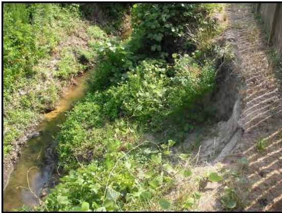
Picture 5-2. Severe bank erosion along landscaping fence
