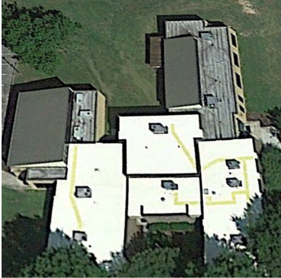
Overview of Roof
