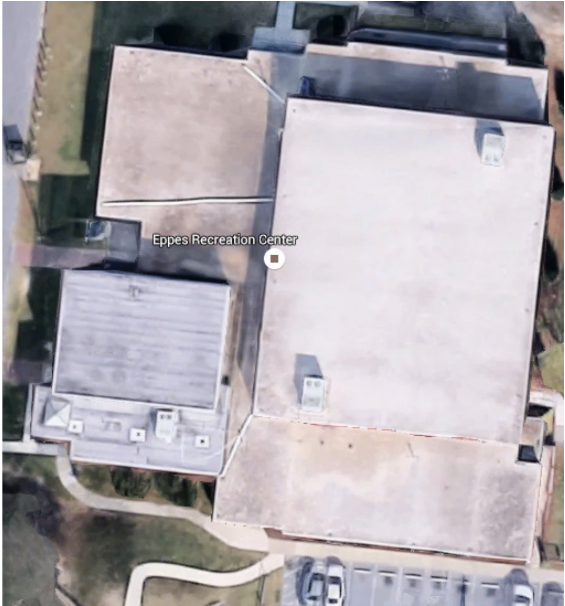
Overview of Roof
