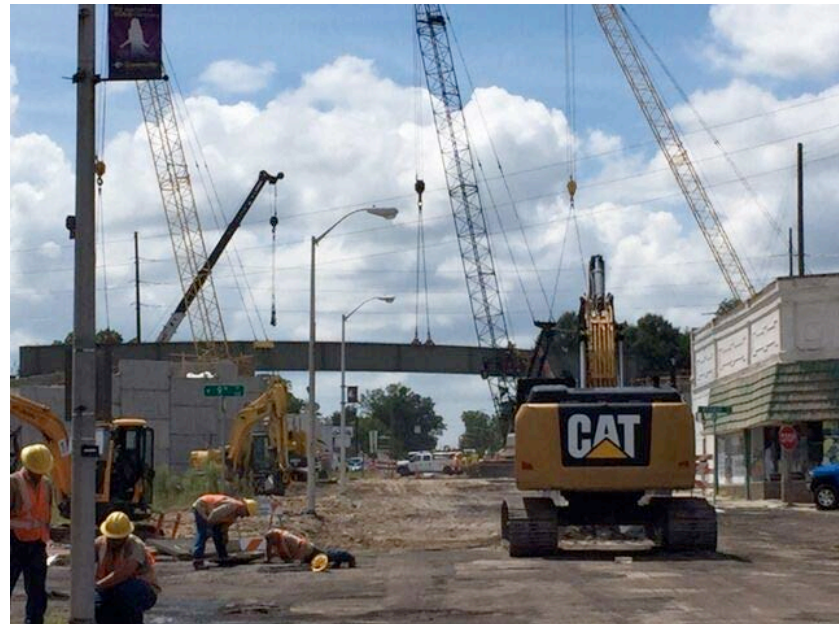
10 th Street Connector Construction
