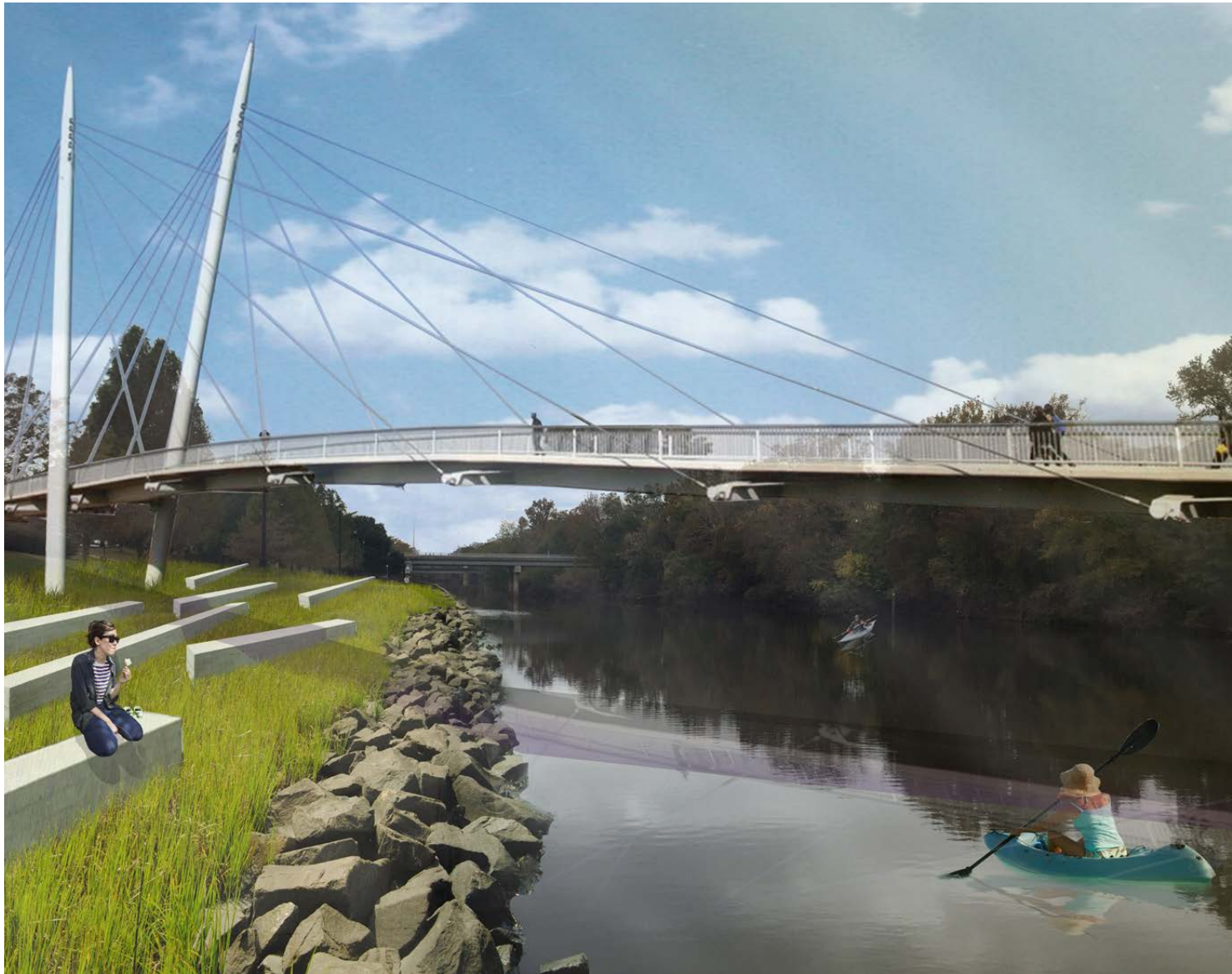
Proposed high visibility iconic bridge and living shoreline, pending hydraulic study, permitting and funding.
