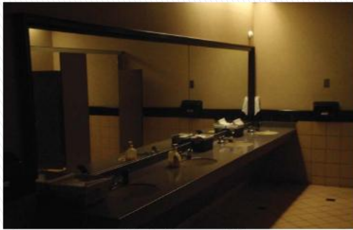
Restrooms - upgrade finishes, partitions, counters and mirrors to match new design
