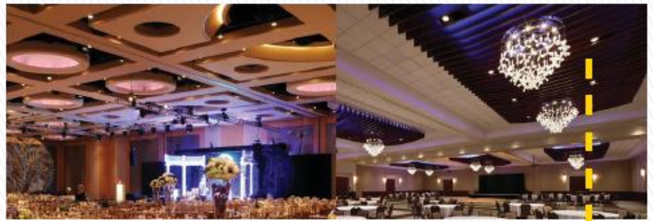
Examples of ceiling panels with multi-function lights
