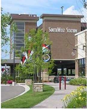
Southwest Station Eden Prairie, MN Architect: not known
