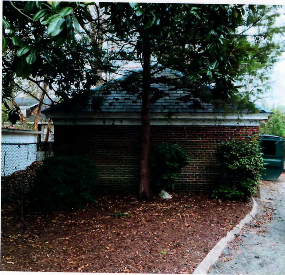
View of garage from south (5 th Street) side.
