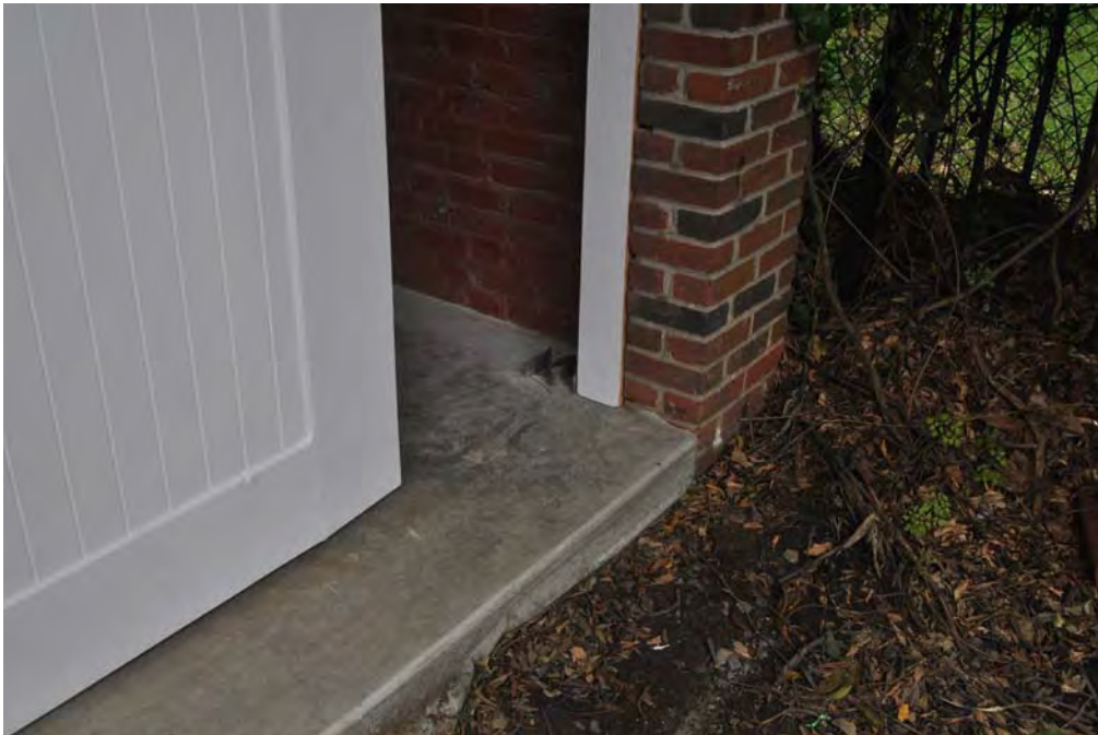
803 E Fifth Street – Concrete floor
