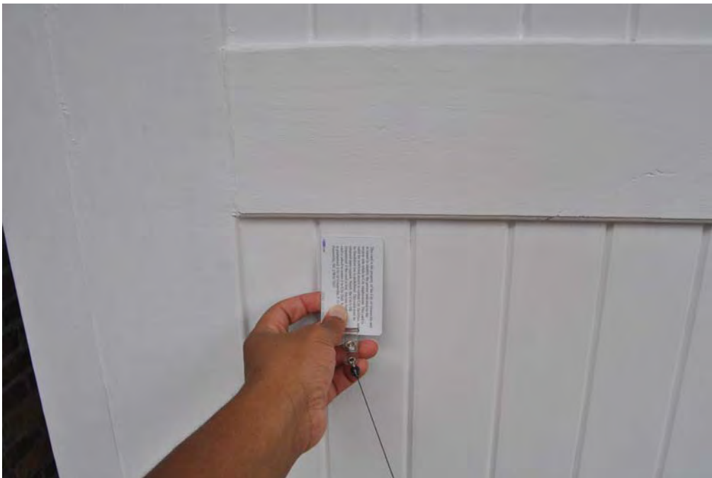
803 E Fifth Street – View of panels
