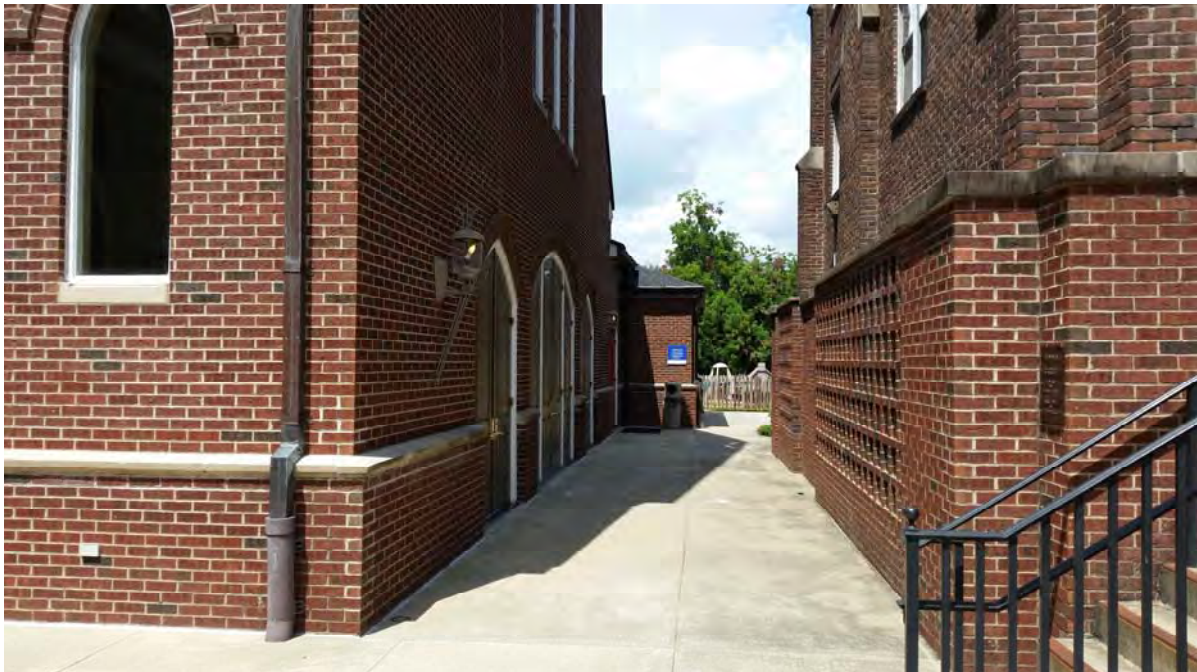
401 E. Fourth Street – View of doors to receive awnings
