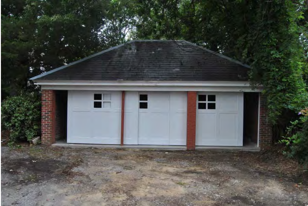
803 E Fifth Street – Front of garage
