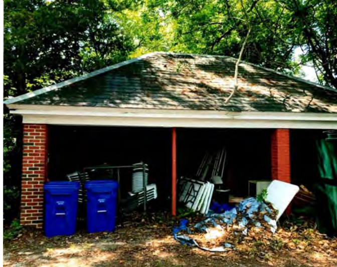
803 E Fifth Street – Front of garage (before)
