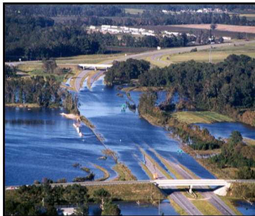
Image 1: Flooded View of Highway 264 Bypass
