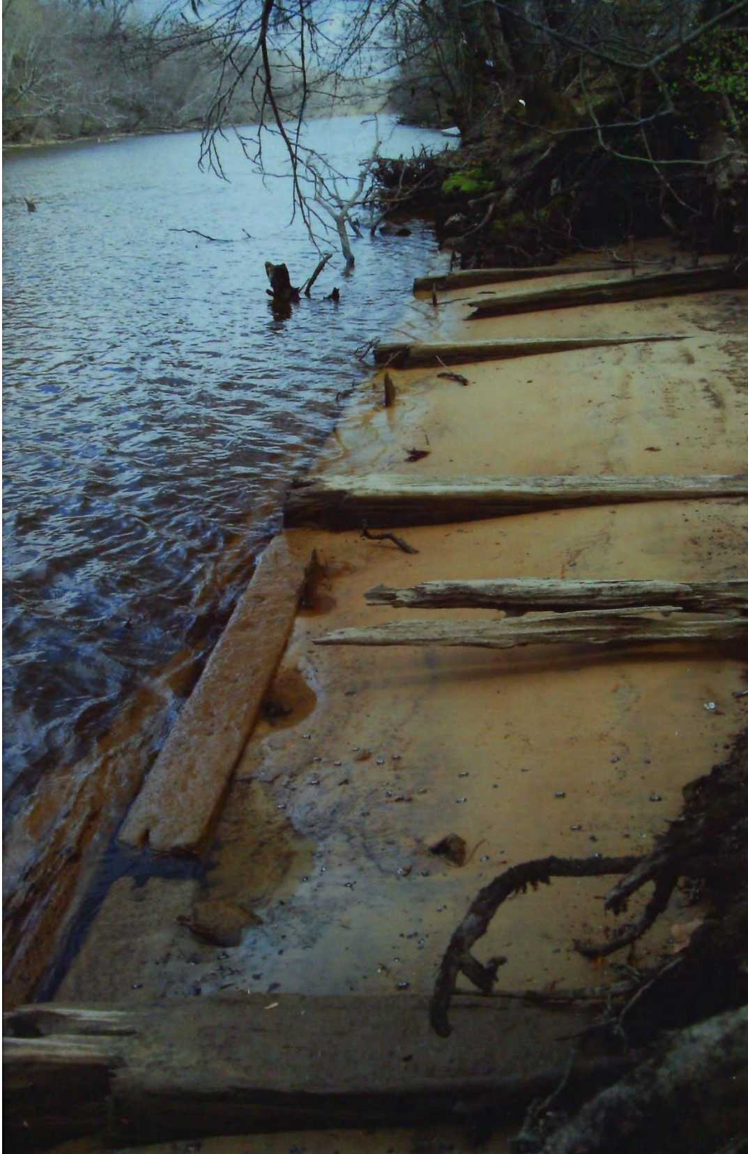
View of Lock Remains Looking East. "East_overallview.jpg" V. Bellis. 2017
