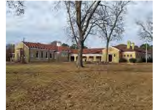
600-700 West Third Street Third Street School & Grounds
