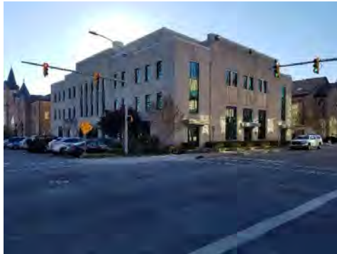
201 West Fifth Street Municipal Building
