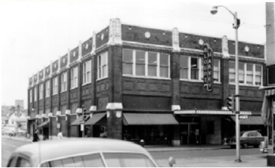
330 Evans Street Blount Harvey Building
