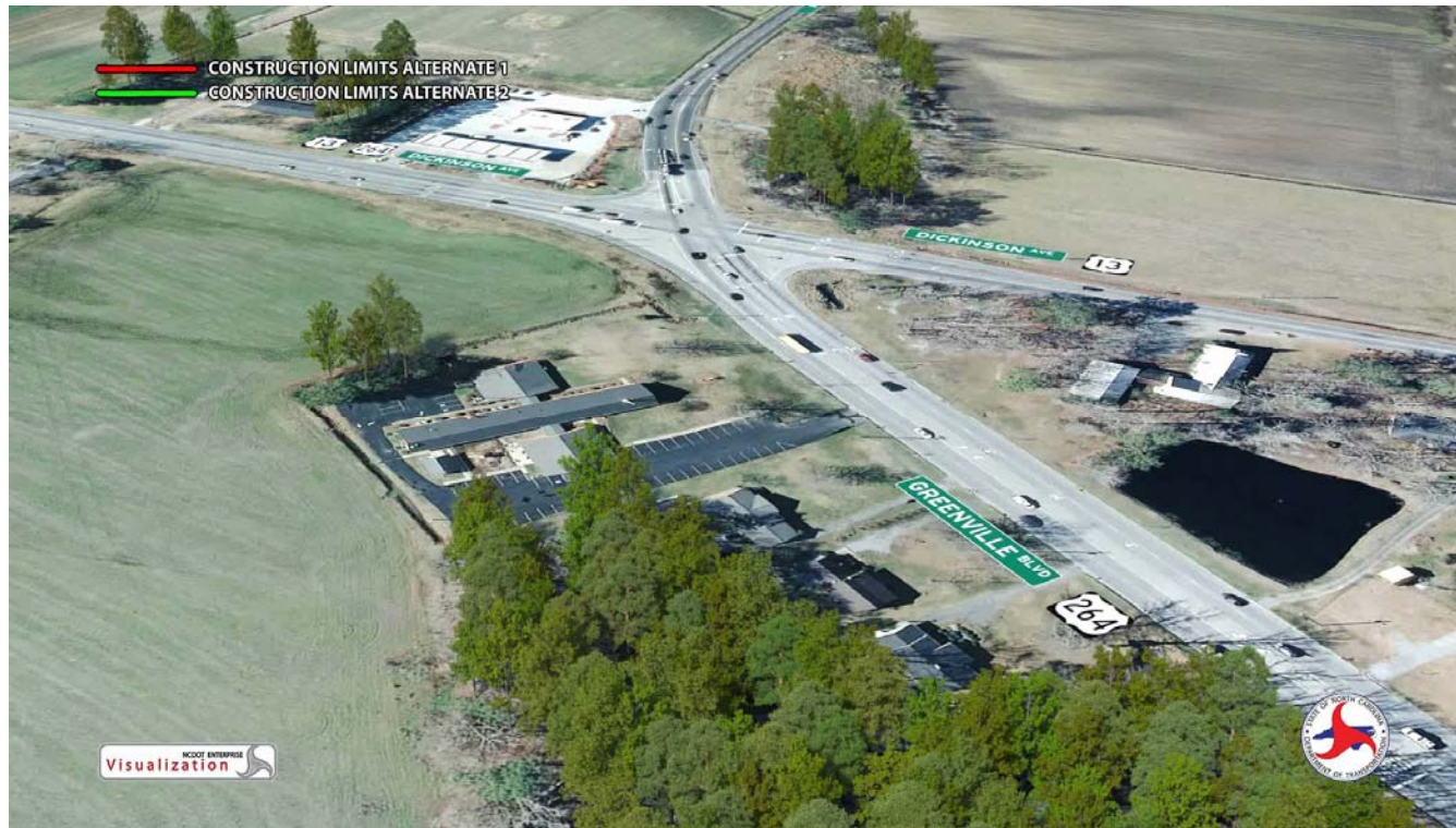
Allen Road Widen to Multi-Lanes (STIP No. U-5875)
