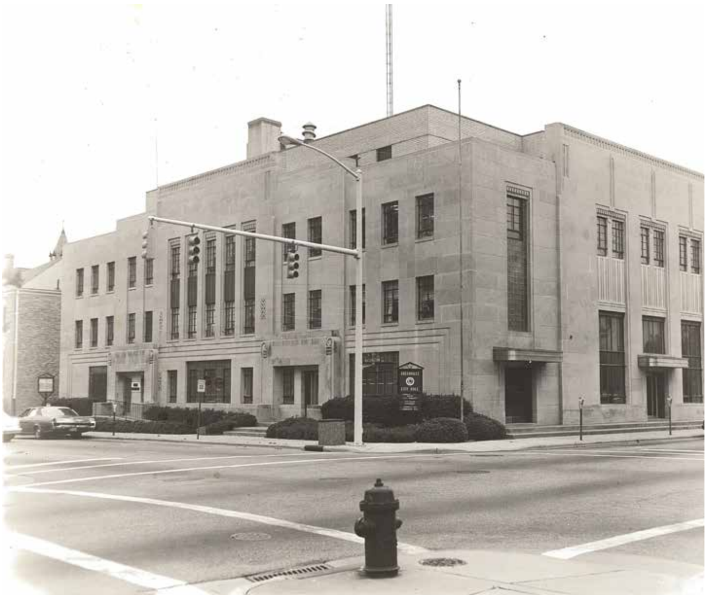
Current Municipal Building - Former City Hall
