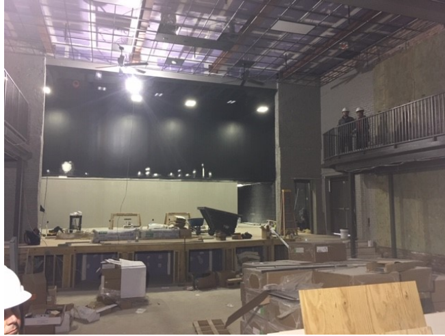
View of stage from left side of building
