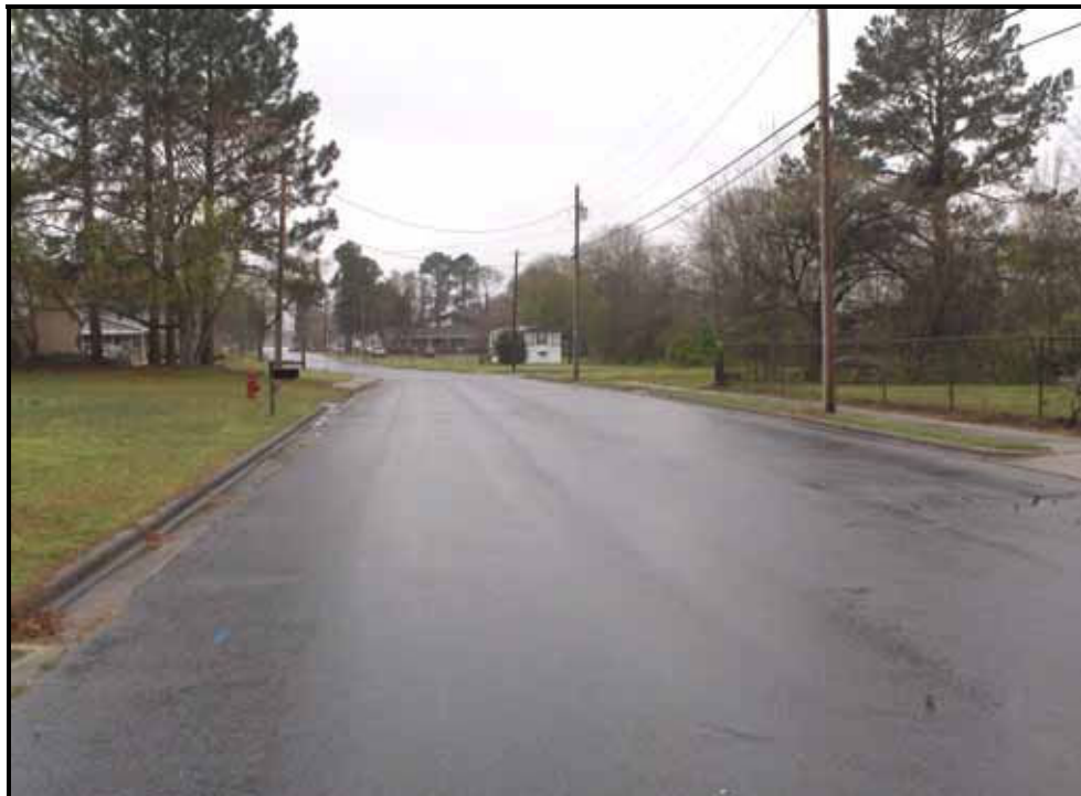
VIEW OF WEST MOORE STREET FACING NORTHWEST
