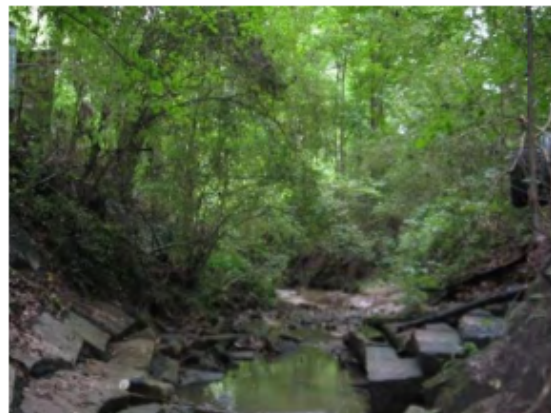
Picture 5-6: Existing Bank Revetments
