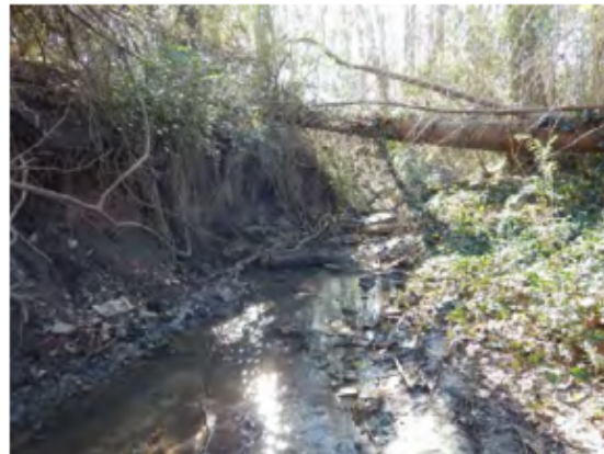
Picture 5-5: Right Stream Bank Erosion
