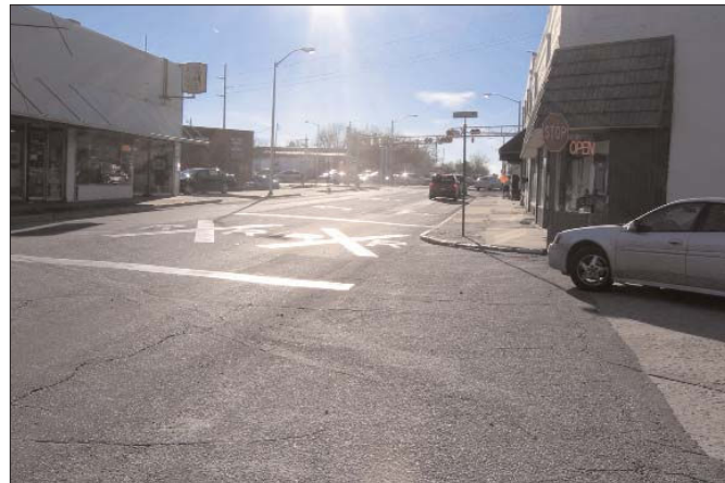
Dickinson Avenue at 10th Street
