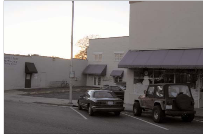
Midblock off-street parking
