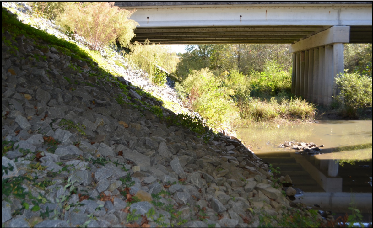
10. Rip rap under Alt 264 bridge
