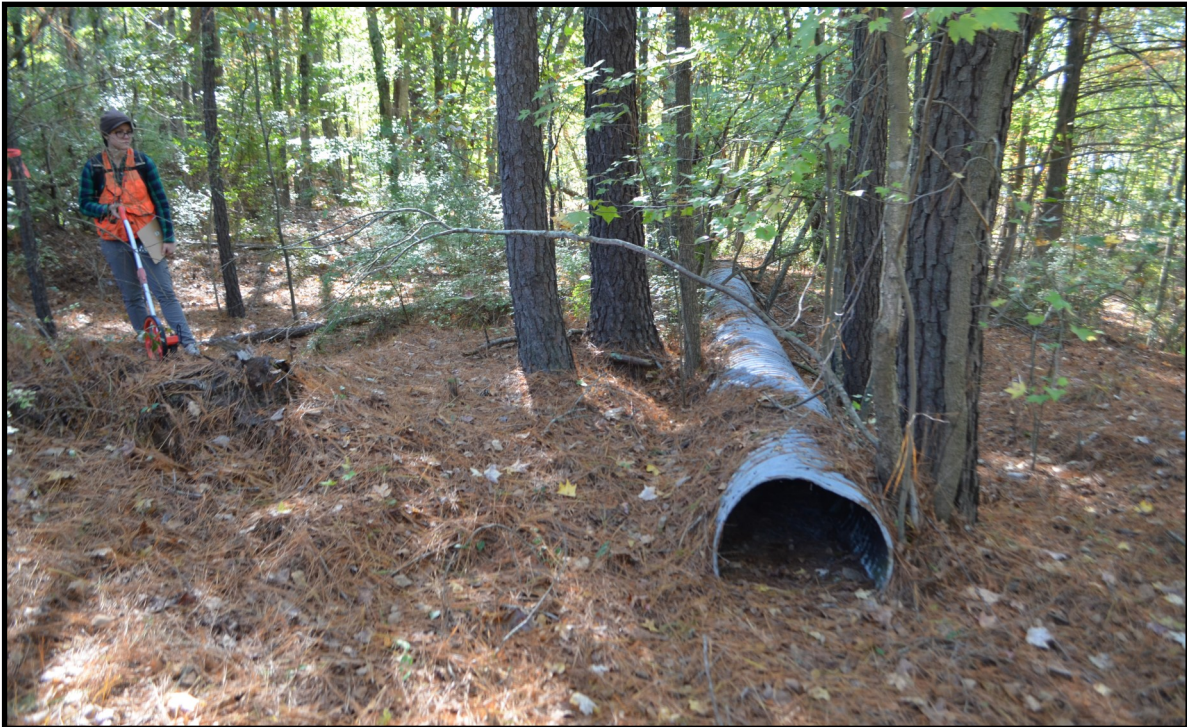
6. Abandoned old culvert along alignment
