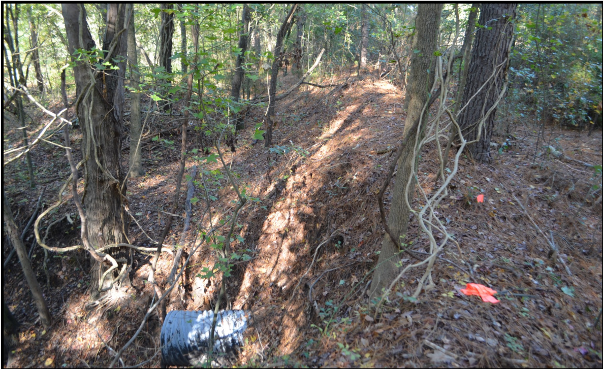
4. Existing culvert crossing
