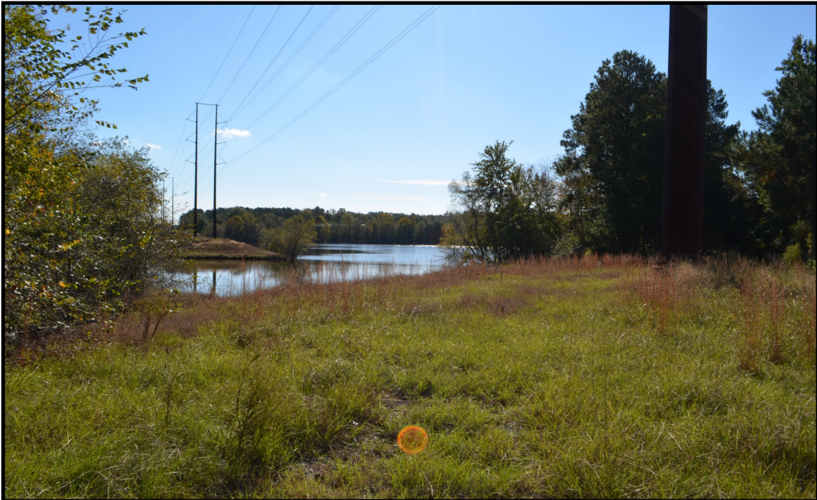
8. Cross power lines on existing grassy road
