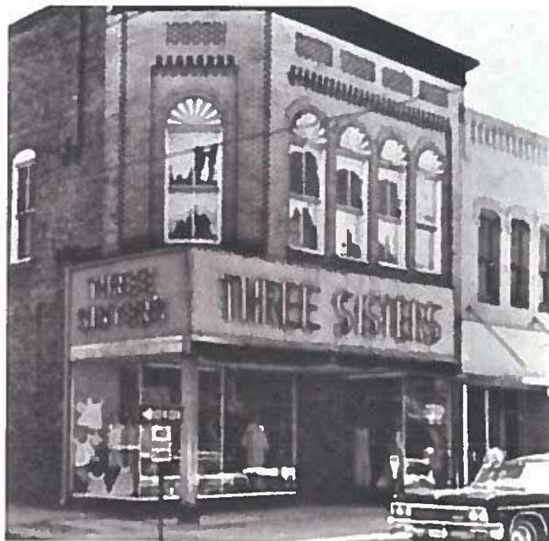
This photograph of the Frank Wilson Store, taken ca. 1968, shows cut back below the front entrance overhang leaving a column and advertising used on the front of the overhang.
