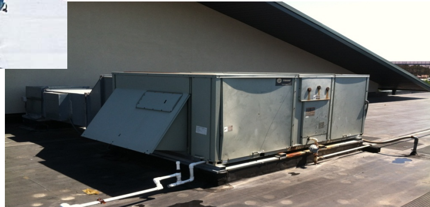
Air Handling Unit Replacement
