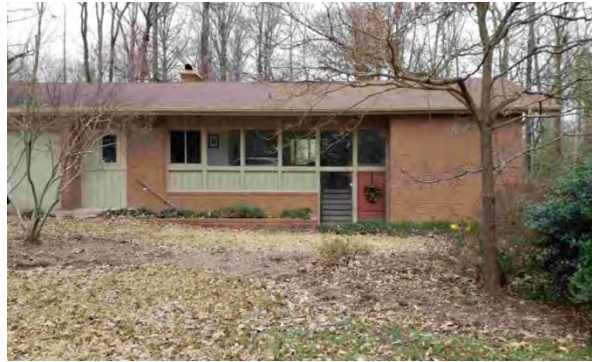
Front entrance below grade
