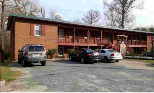
Living units below grade
