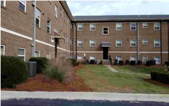
Below grade apartments
