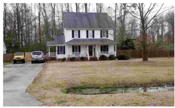
Guttering on lower level
