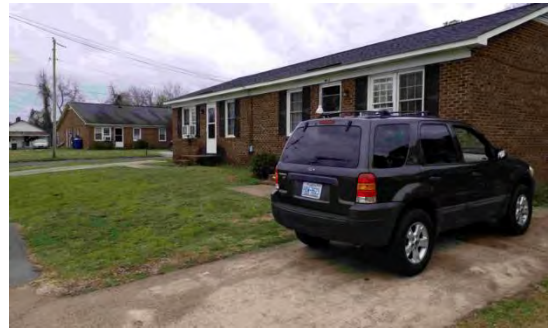
Window unit HVAC system
