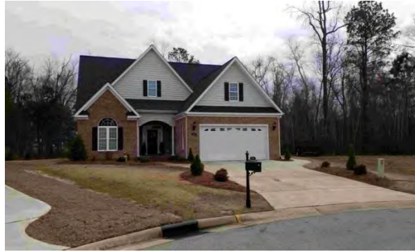
Guttering goes under grade and storm drain at street
