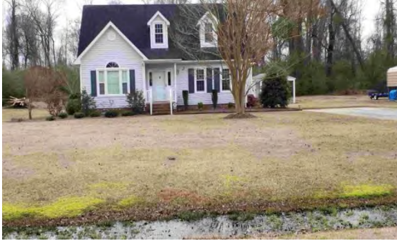
Standing water in drainage ditch
