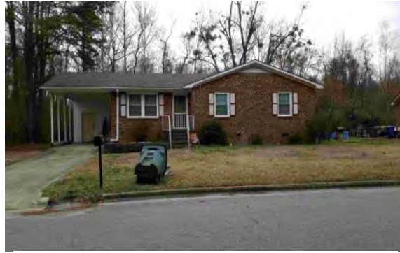
Guttering drains onto driveway
