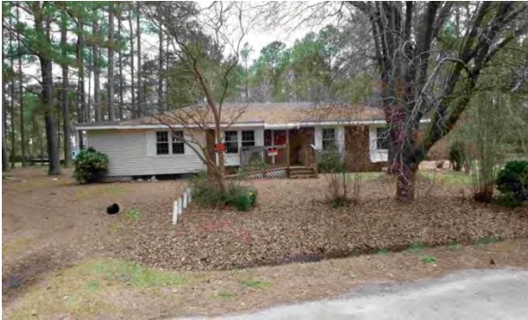
Drainage ditch in front
