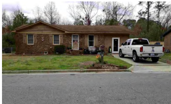
Garage converted to living space and not elevated
