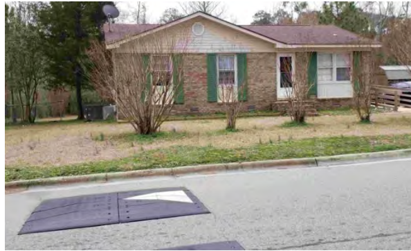
HVAC not elevated on left side of home
