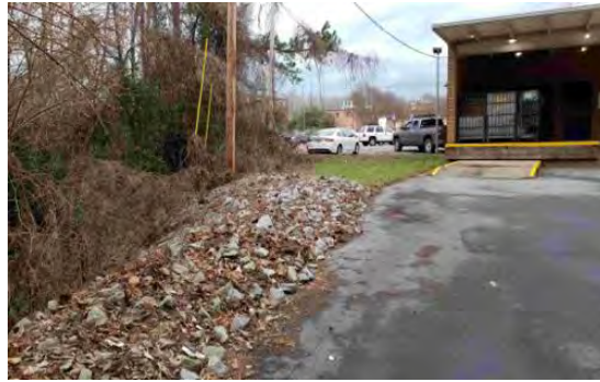
Creek in rear of building
