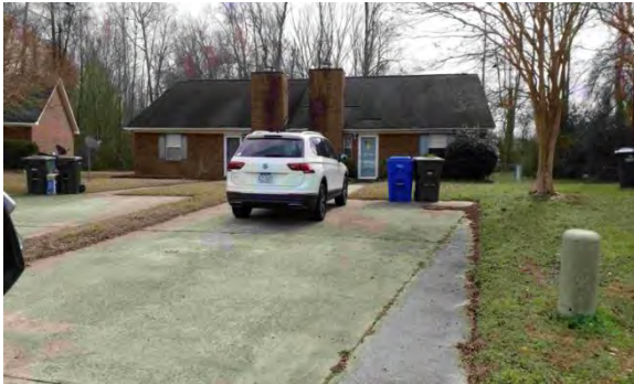
Drainage inlet out front
