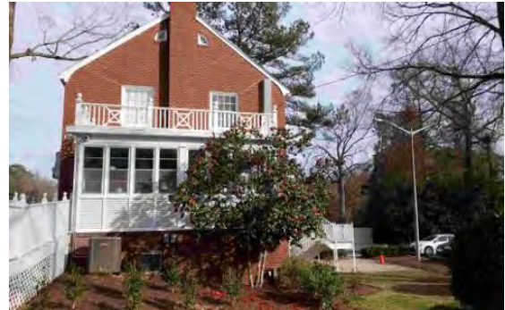
HVAC not elevated
