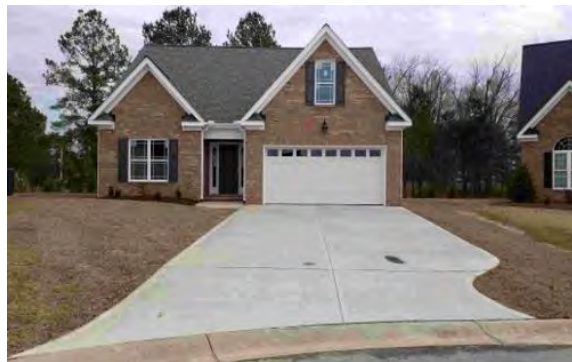
Guttering in front of house under construction
