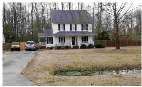
Guttering on lower level
