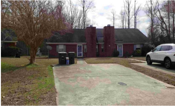
Building sits at lowest point of neighborhood
