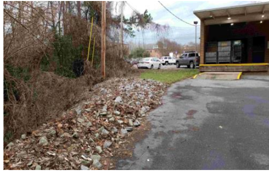
Creek in rear of building
