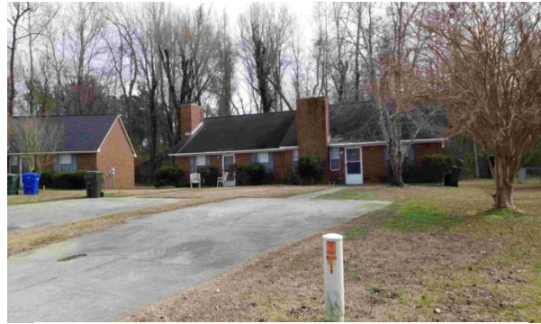
Building at lowest end of neighborhood
