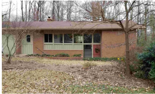
Front entrance below grade
