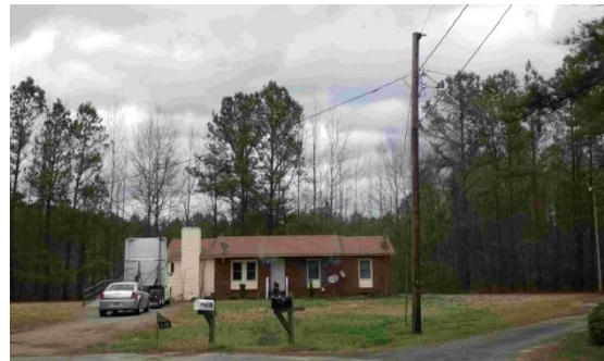
Neighborhood sits several feet below main road grade
