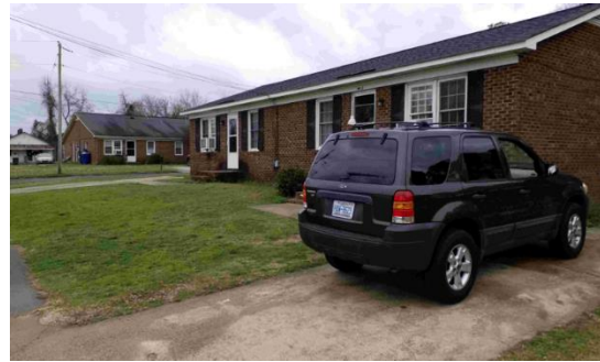
Window unit HVAC system
