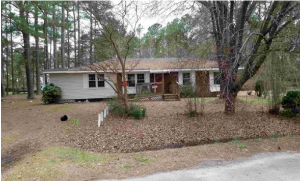
Drainage ditch in front
