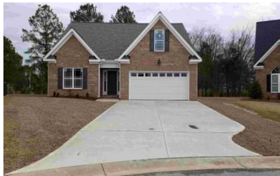
Guttering in front of house under construction
