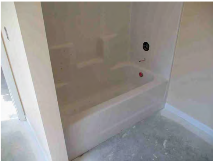
Additional view of master bathroom
