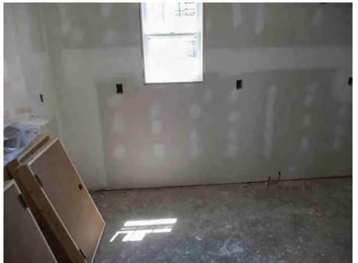
View of kitchen
