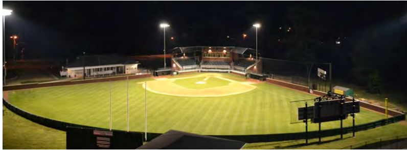
Elm Street Park – Nighttime
