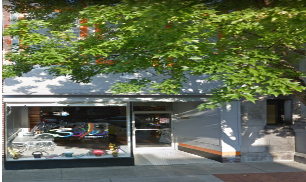
415 Evans Street located in Uptown Greenville.
