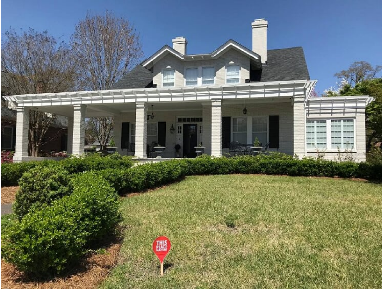
Fig. 1: Front Façade of House
