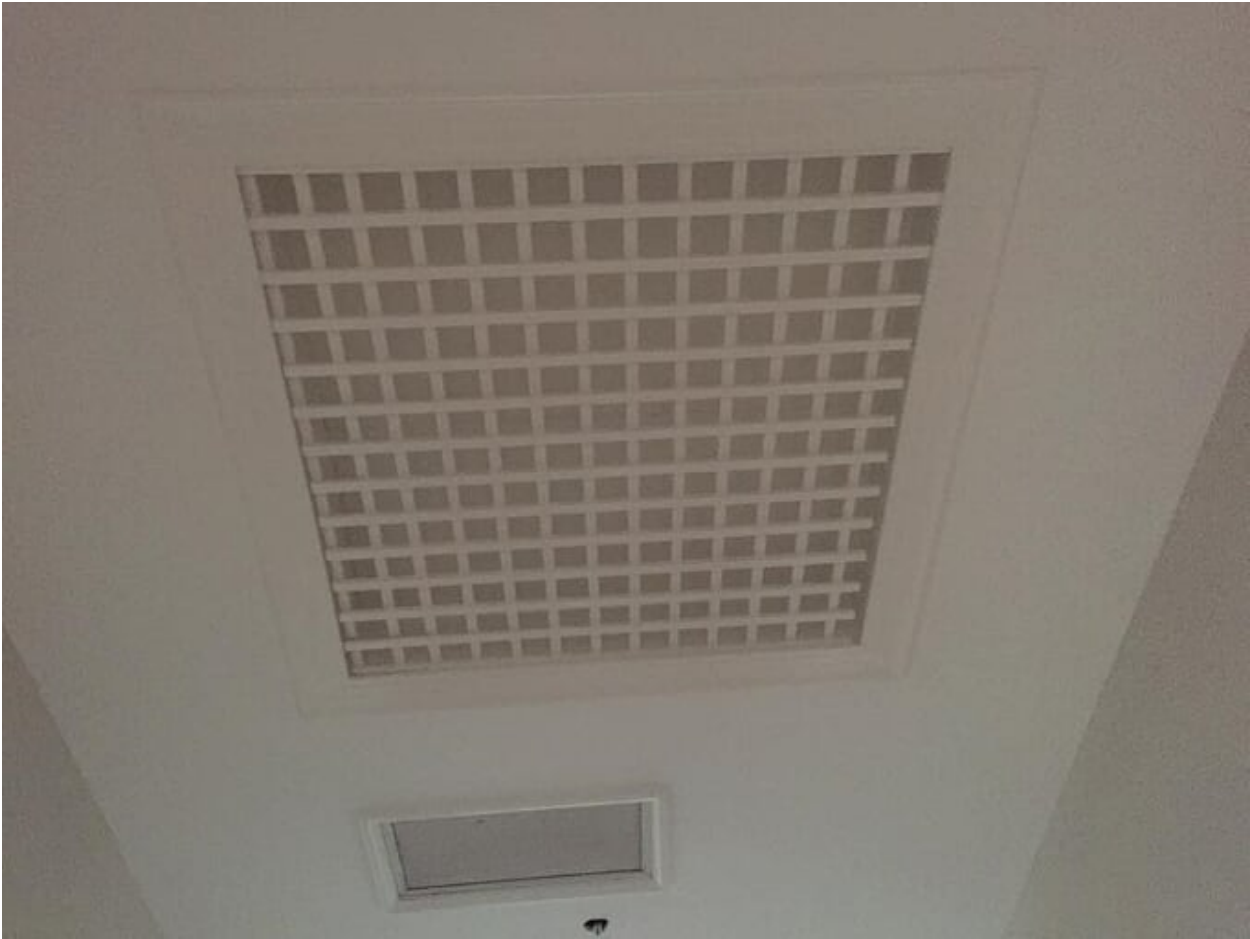
Fig. 19: Photograph of Original Attic Fan Vent Grill in Upstairs Ceiling
