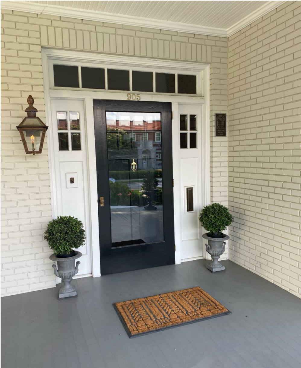
Fig. 6: Photograph of the Exterior of the Front Door
