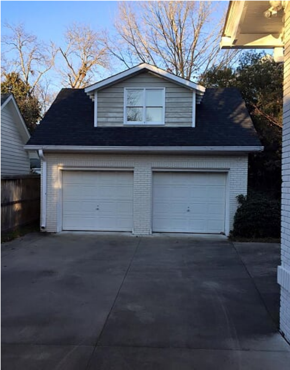
Fig. 7: Exterior Façade of the Garage
