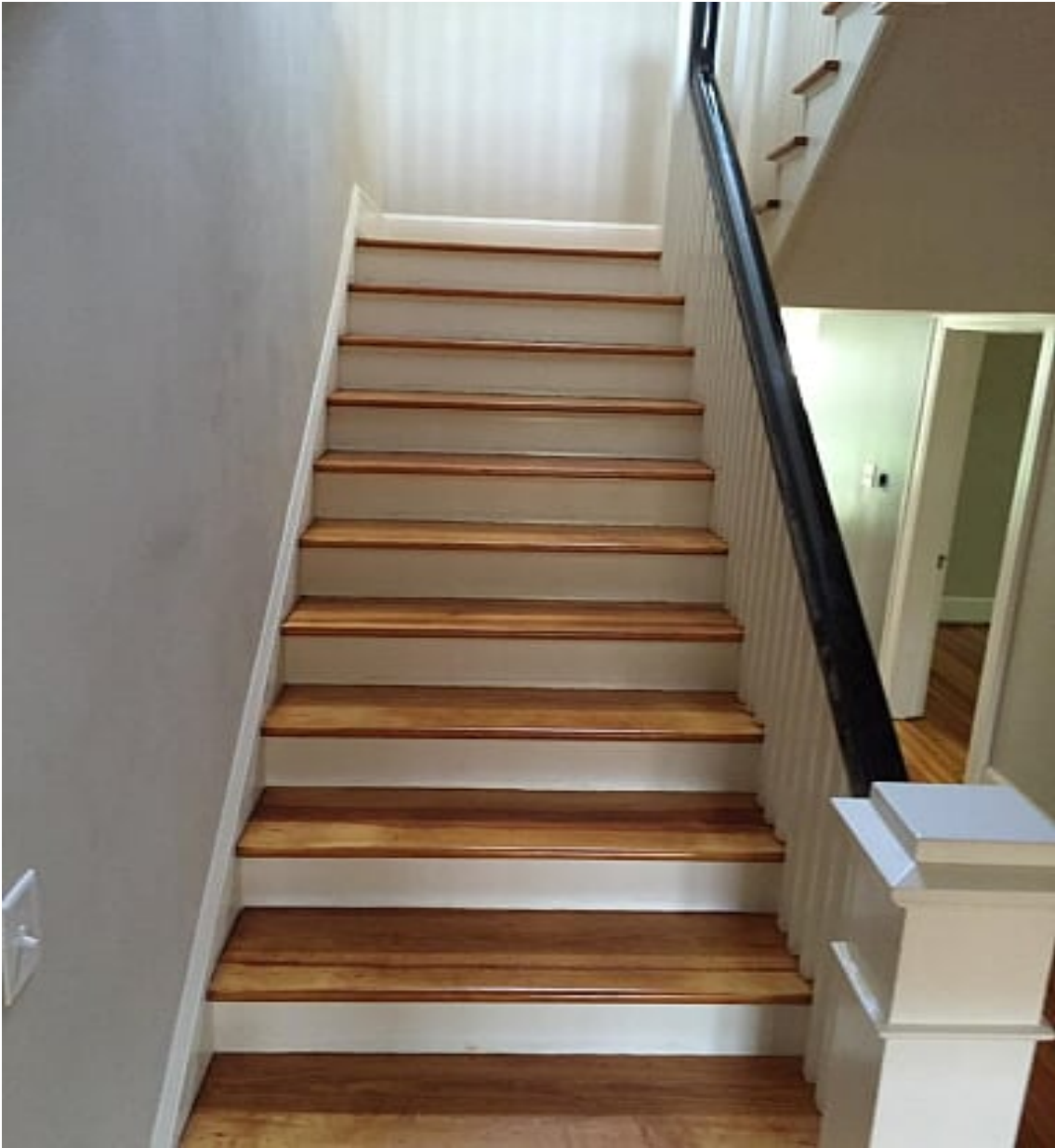
Fig. 16: Photograph of the Staircase Looking Upstairs
