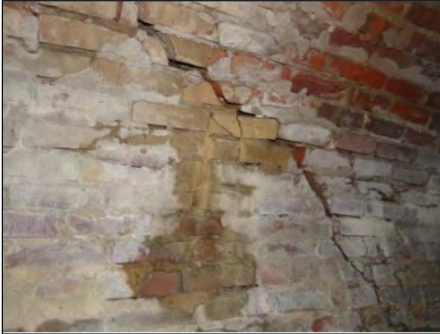
Photo 3: Brick Arch with Cracks
