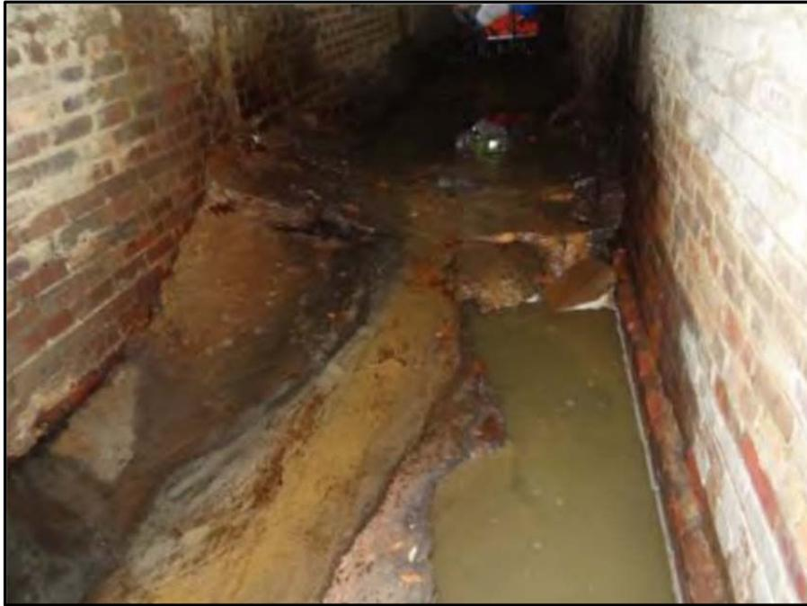
Photo 1: Floor Heaving and Cracking
