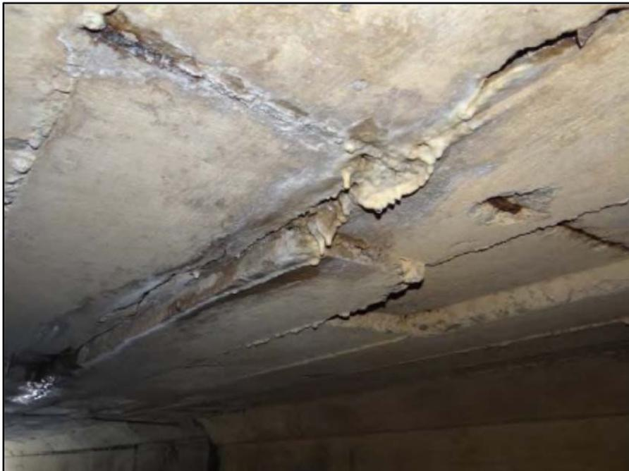
Photo 4: Concrete Box with Spalling and Exposed Steel
