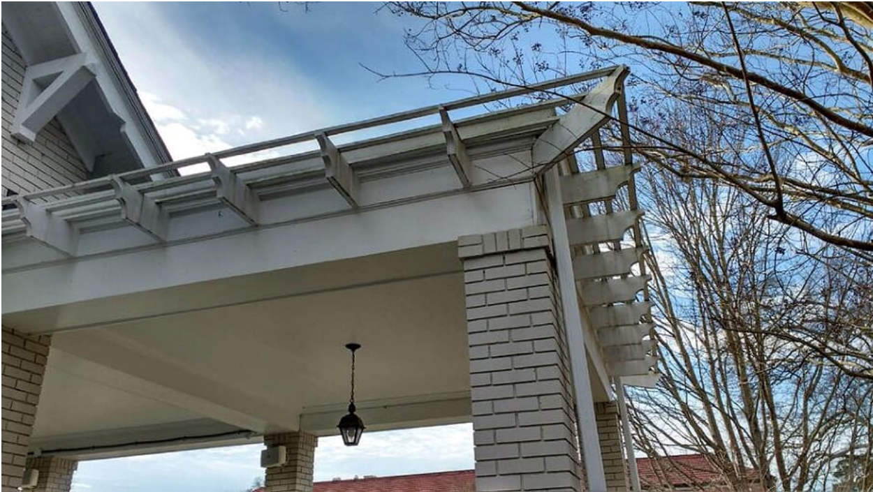
Fig. 5: Detail of the Overhang on Porch-cochere
