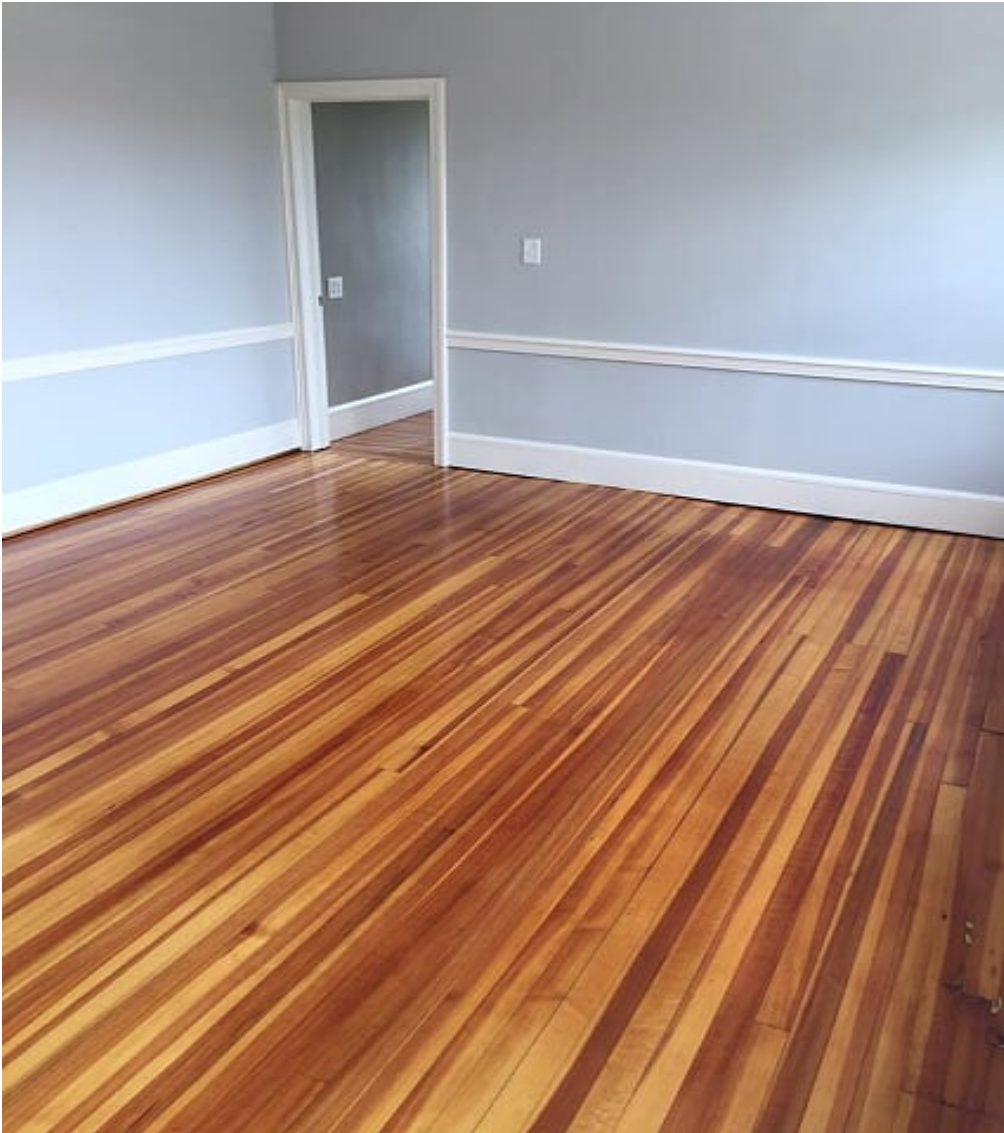
Fig. 18: Photograph of Floor of the Master Bedroom Upstairs
