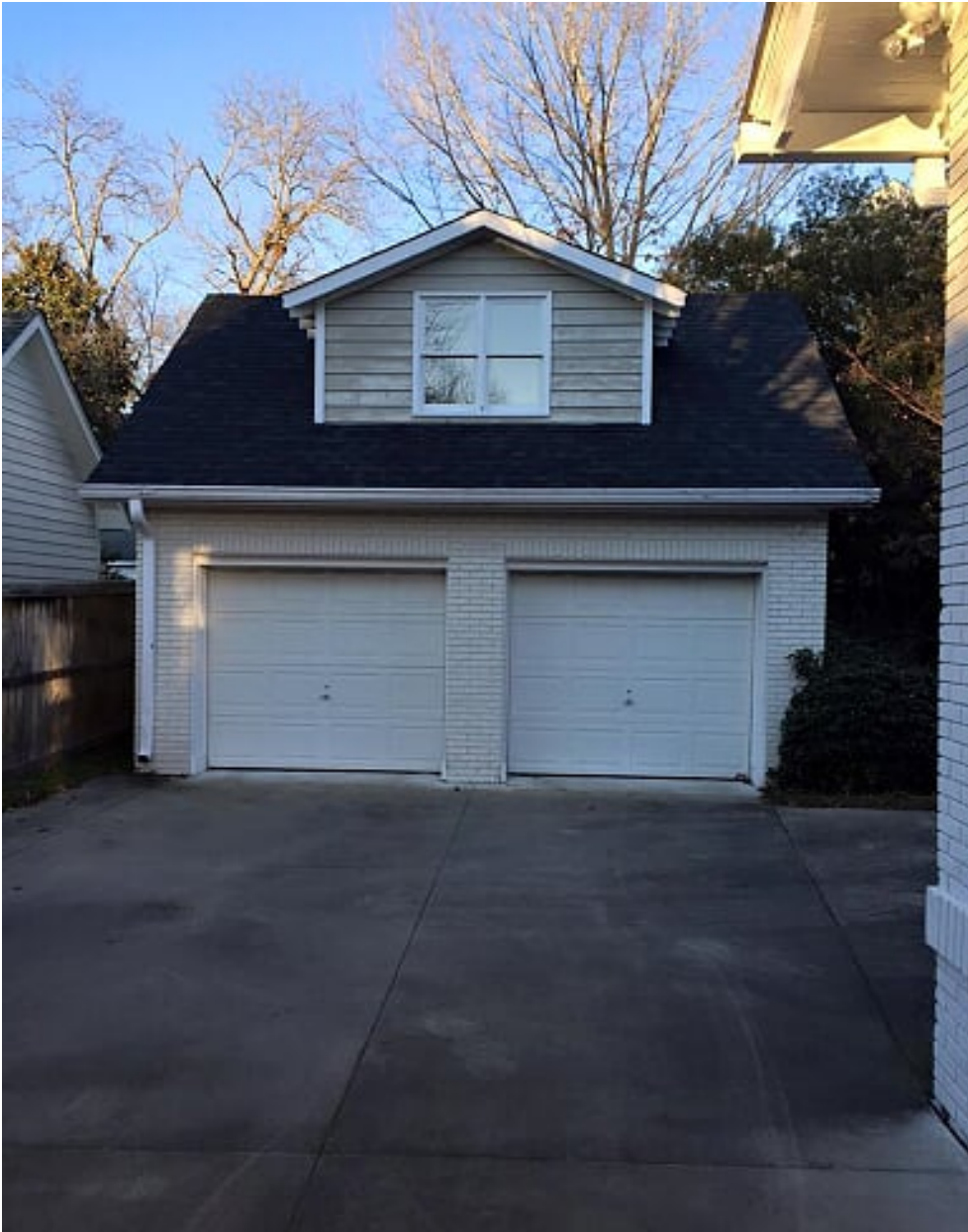
Fig. 7: Exterior Façade of the Garage
