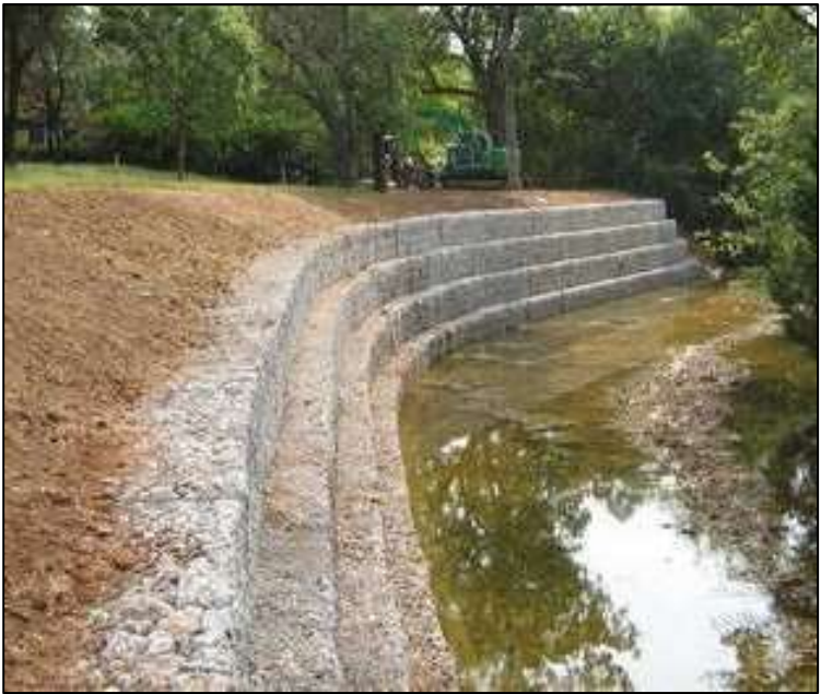
Example of gabion retaining wall for streambank stabilization.
